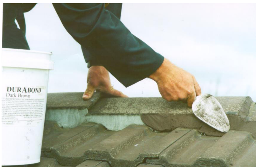
Application of DurAbond™ Roof Pointing Compound
