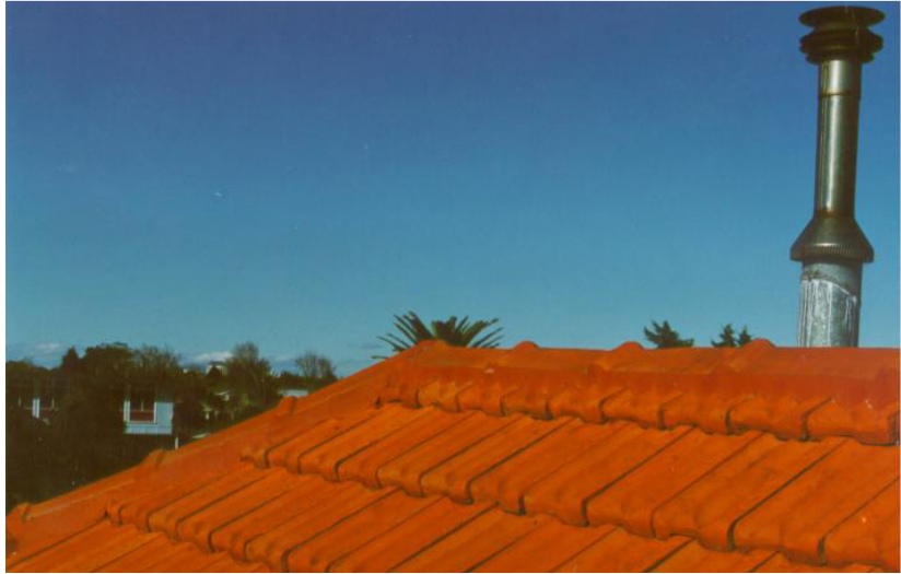
Completed DurAbond™ Roof Pointing Compound
