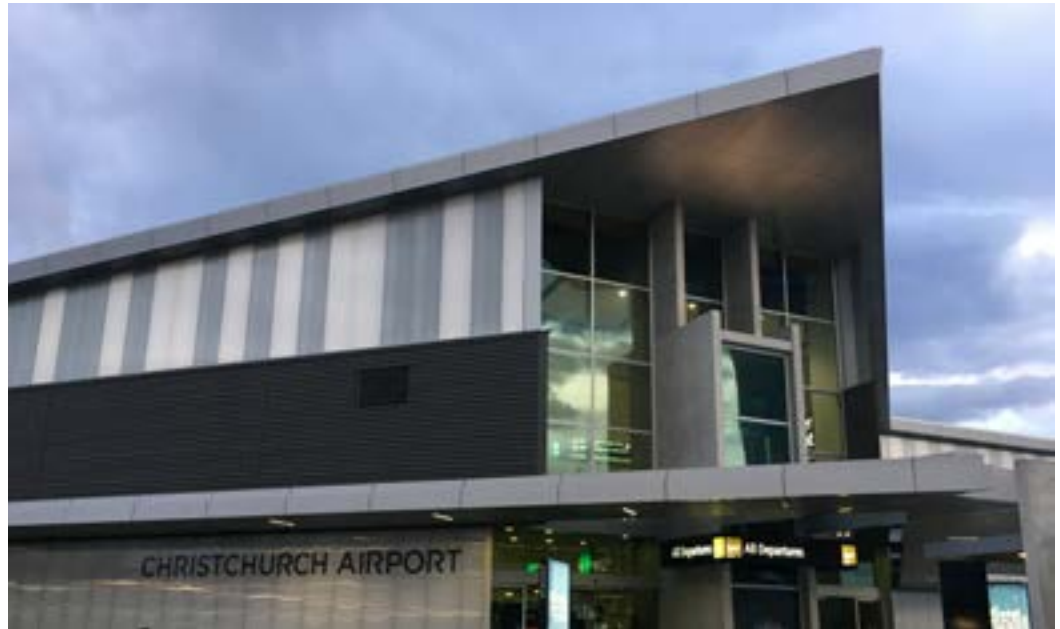
Christchurch International Airport 4500 m 2 of 1.5 mm Grey Butynol used for flat roof areas and gutters. Completed in 2013.
