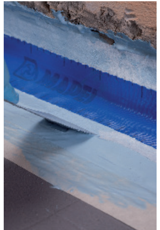
Application of Mapeband to a wall-floor joint with Mapelastc AquaDefense
