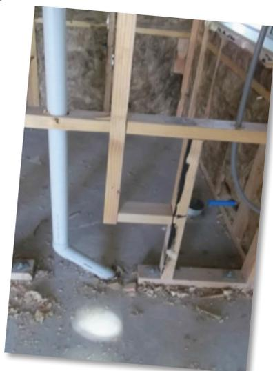
A large cut-out that the builder said would be repaired (but repairs are unlikely to be adequate due to the geometry). Appears to be a bracing wall re HD bolts.
