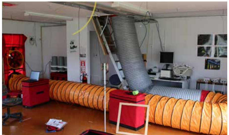
The dual fan method used to assess airtightness in roof cavities. The top fan in the door blows air into the living space while the bottom fan and ducting move outside air into the roof space.
