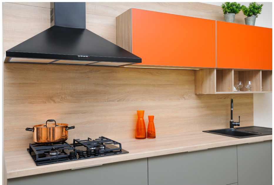
Cooking generates large amounts of moisture and particles that cannot be removed by passive ventilation alone. Kitchens, bathrooms and laundries should have localised extractors to remove moisture at source.
