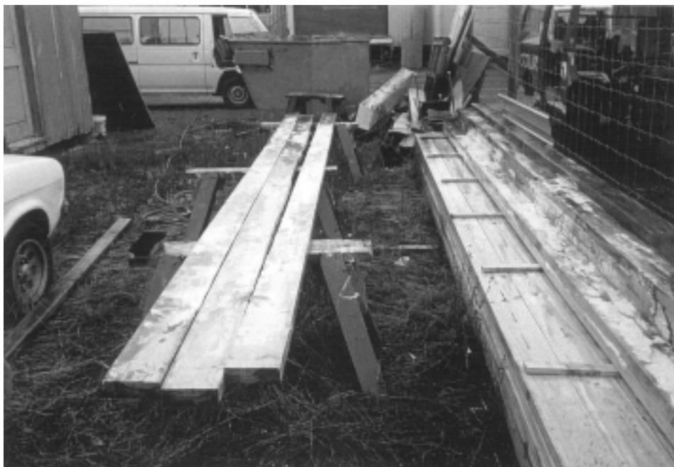
Rot showing on timber that has been stored outside for a long period and moisture has penetrated the protective covering.
