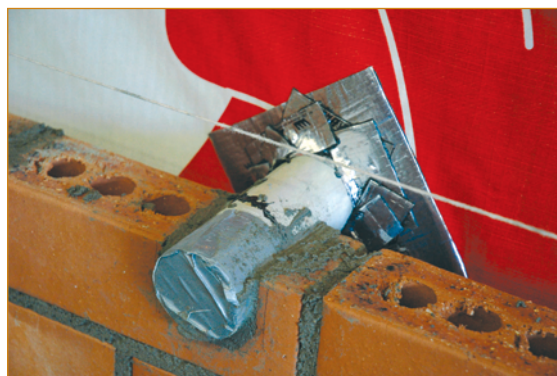
Figure 10: Penetration detailing showing taping to the wall underlay.
