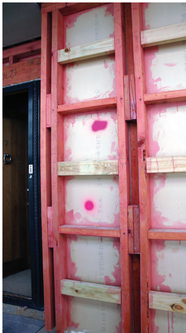
Figure 2 Timber in external walls that is sound but untreated (or not treated to current B2/AS1 requirements) should be given two coats of brush-on boron glycol preservative treatment as part of any remediation work
