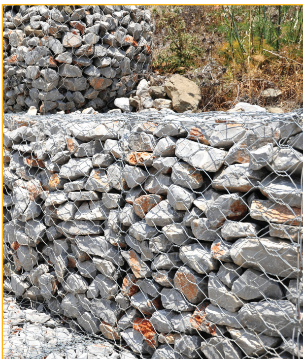
Low gabion wall.
