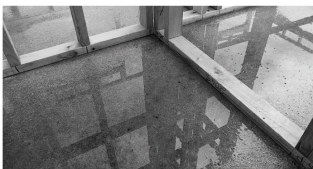
Wet flooring and bottom plates.
