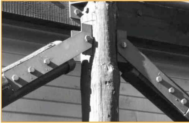
Pole braces with non-adjustable metal brackets.
