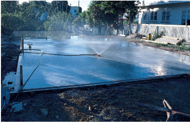
Figure 3. Curing concrete using a fine mist sprinkler.
