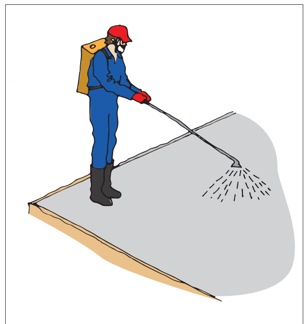
Figure 4. Curing compounds are spray applied.
