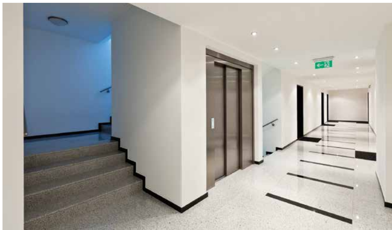
A lift is a specified system and requires regular inspections and maintenance.
