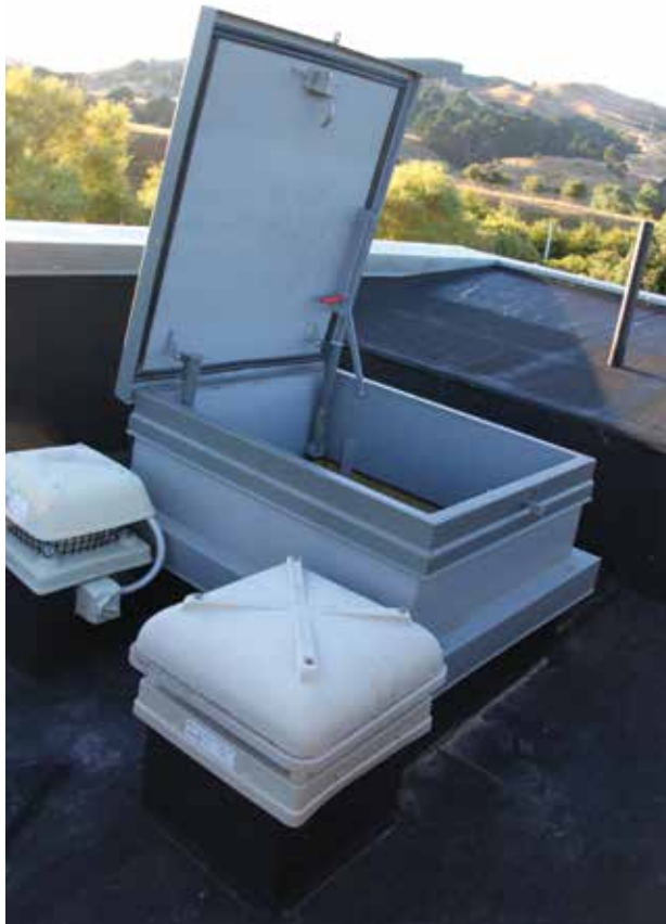
Proprietary roof hatch to provide waterproof, secure and safe roof access.
