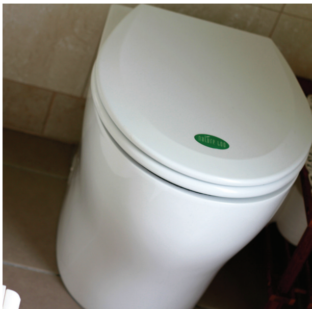
Pedestal for a split-system composting toilet where collection/treatment chambers are located below the bathroom floor.
