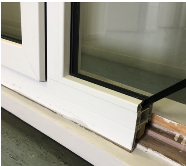
Figure 8. uPVC frames with IGU retrofitted into timber window.
