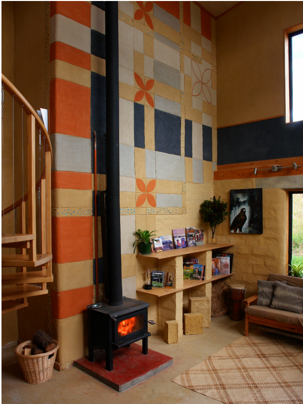
Colours and textures can be added using pigments and minerals in earthen plasters.
