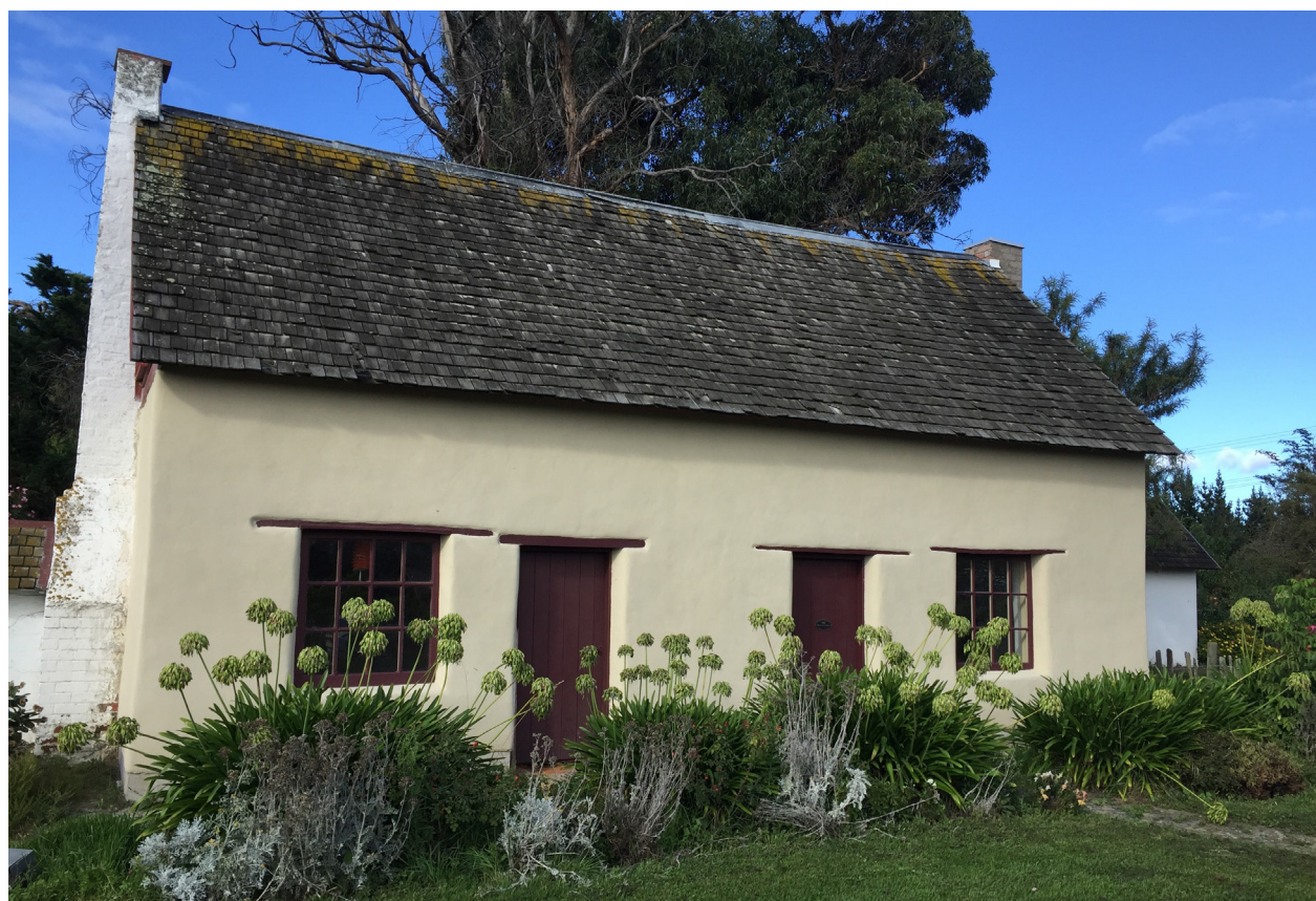
Figure 1. Earth building has a long track record in Aotearoa New Zealand. This cob cottage in Marlborough was built around the early 1860s and restored in the 1960s.
