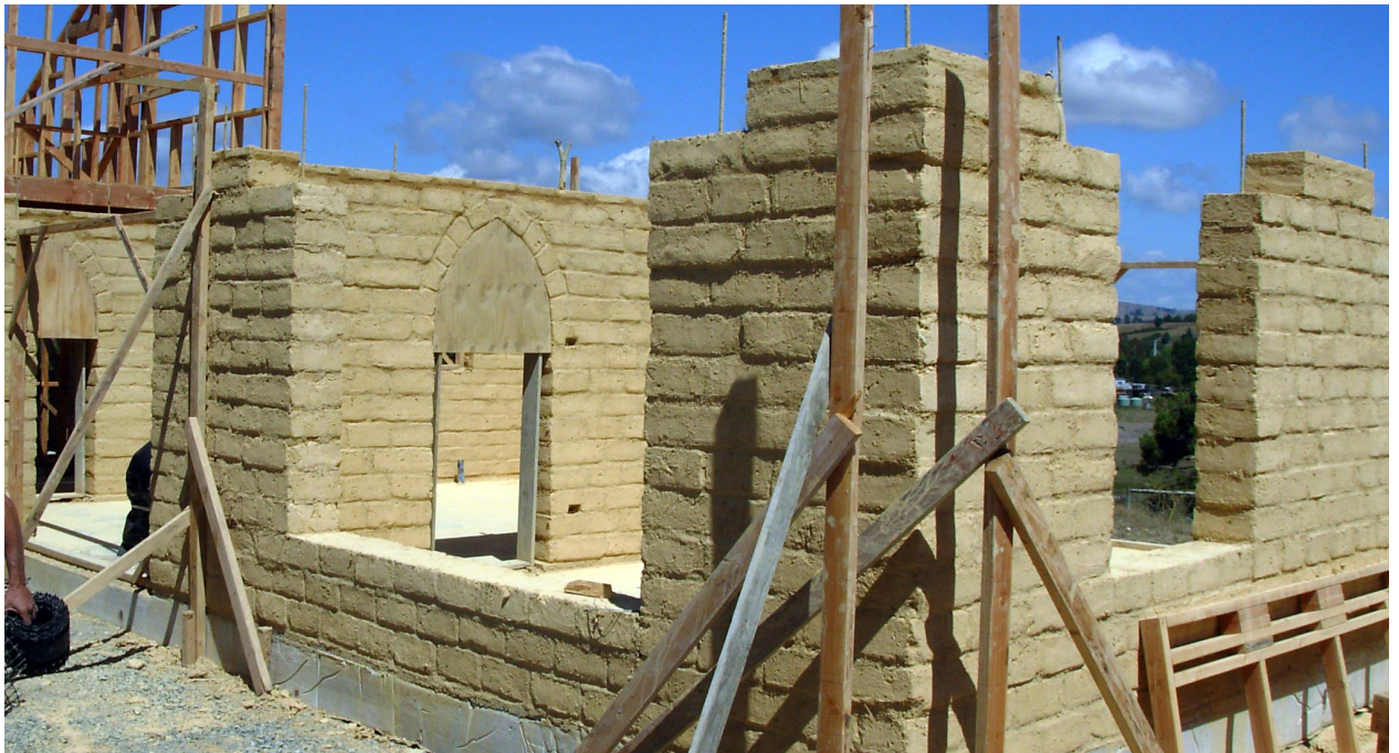
Adobe/mud brick walls under construction.
