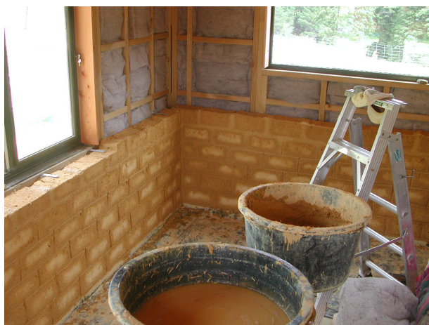
Figure 2. Adobe brick veneer being added to an interior wall.
