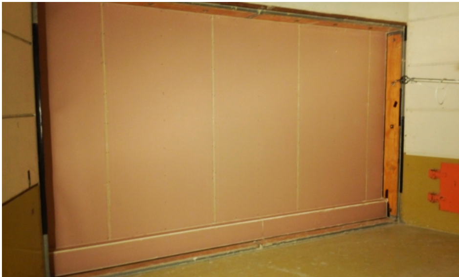
Figure 22. Our test wall built into the acoustic chambers' test aperture.
