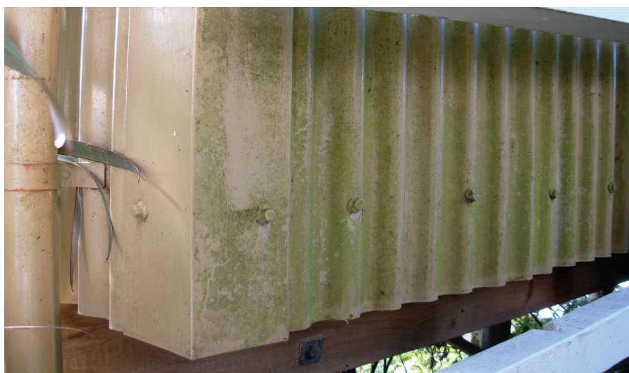
Figure 3. Coatings such as paint must be kept in good condition to remain effective. The mould growth here indicates insufficient maintenance.
