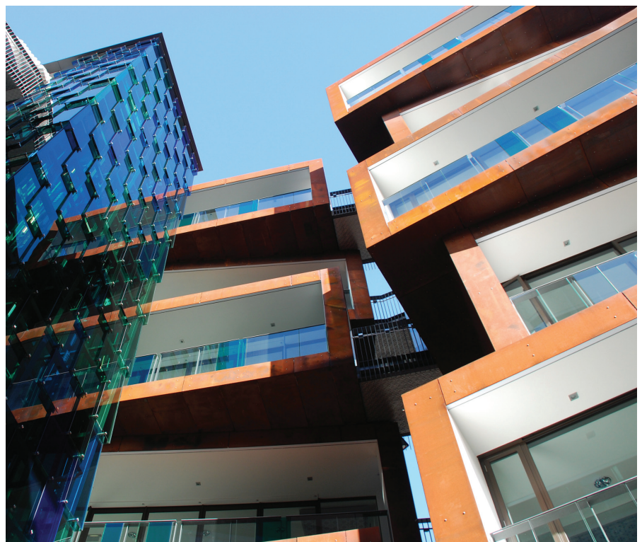
Figure 1. The Ironbank building in central Auckland features weathering steel facades.
