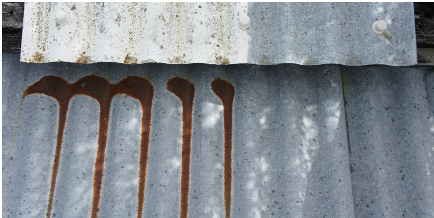
Figure 4. Corrosion of galvanized steel induced by water run-off from a painted galvanized steel surface.
