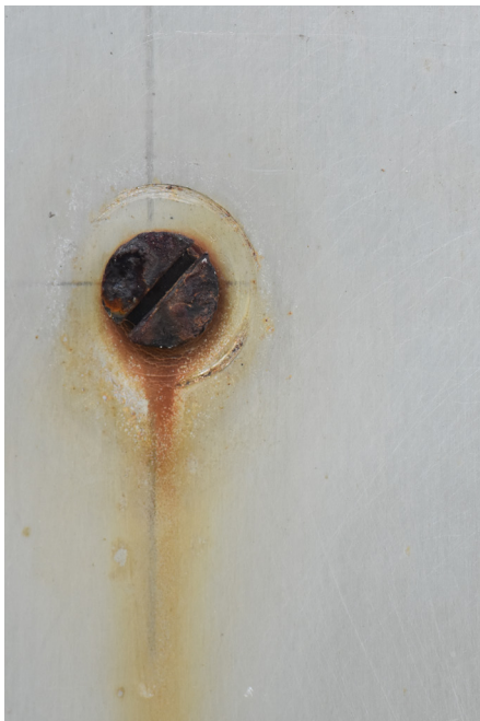
Figure 5. The appropriate level of corrosion protection for different environments is given in documents such as NZS 3604:2011.
