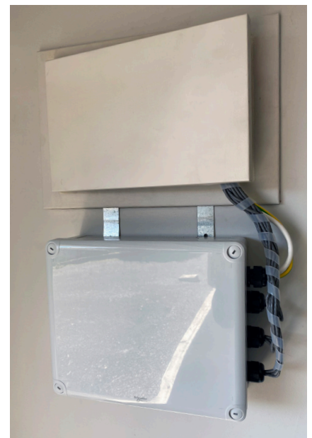
The IoTaWatt™ is contained in a specially made box and mounted next to the switchboard.
