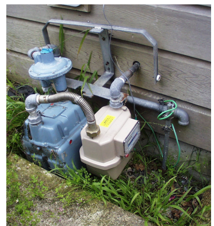
BRANZ gas meter installed side by side with existing meter (picture is from HEEP1).
