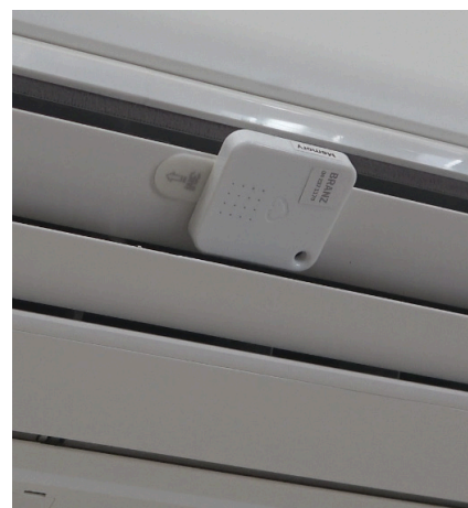
Wireless tags can be mounted on a heat pump to measure temperature close to the source.
