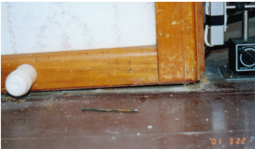
Figure 32: Upper floor skirting board lifting
