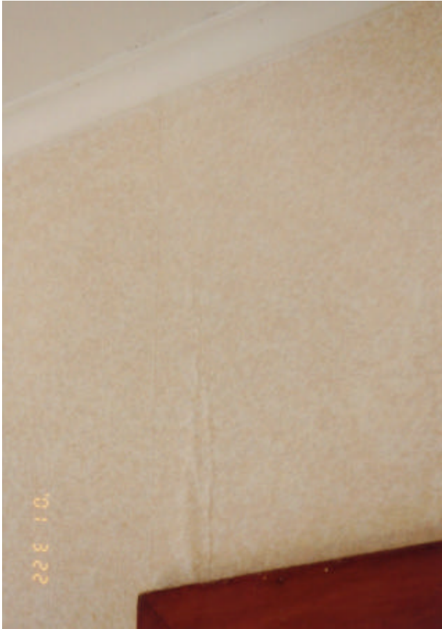
Figure 31: Wallpaper concertinaing under racking load
