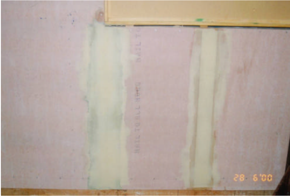
Figure 8: Repaired fibre cement board joints on left side
