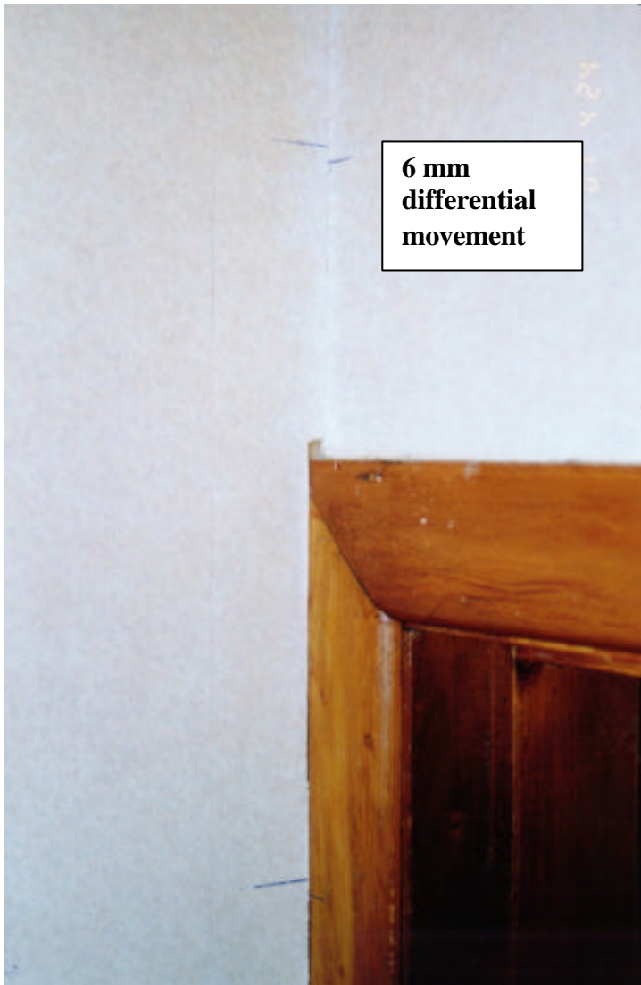
Figure 40: Differential movement between the test wall and the transverse hall wall
