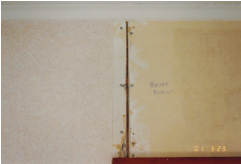
Figure 33: Prepared gypsum plasterboard joint ready for re-stopping
