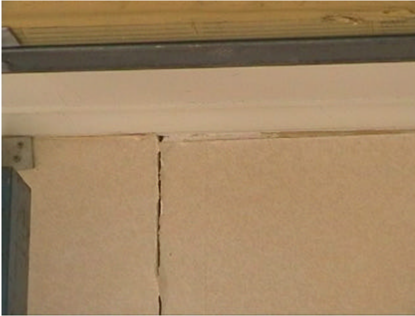
Figure 43: Shear slippage between lining sheets in lounge
