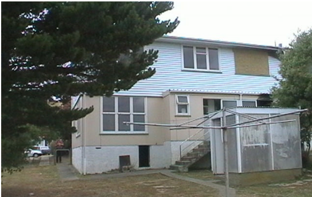
Figure 26: Back view of test house
