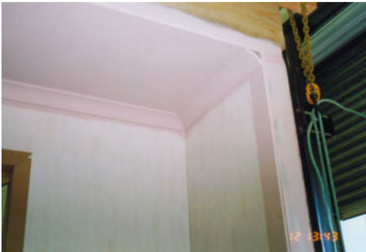
Figure 4: Section of ceiling and walls complete with cornice in place
