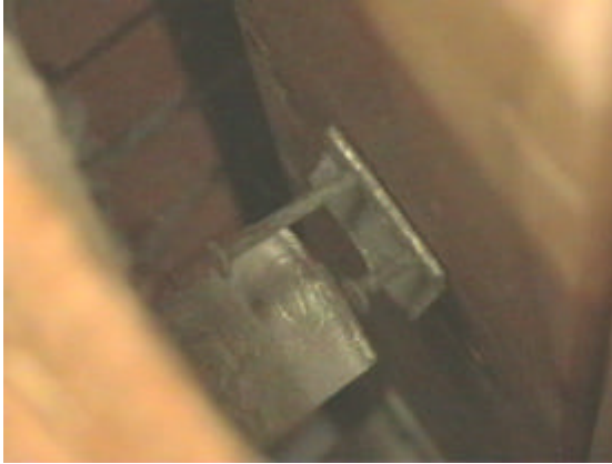
Figure 23: Nails pulled from frame and tie broken
