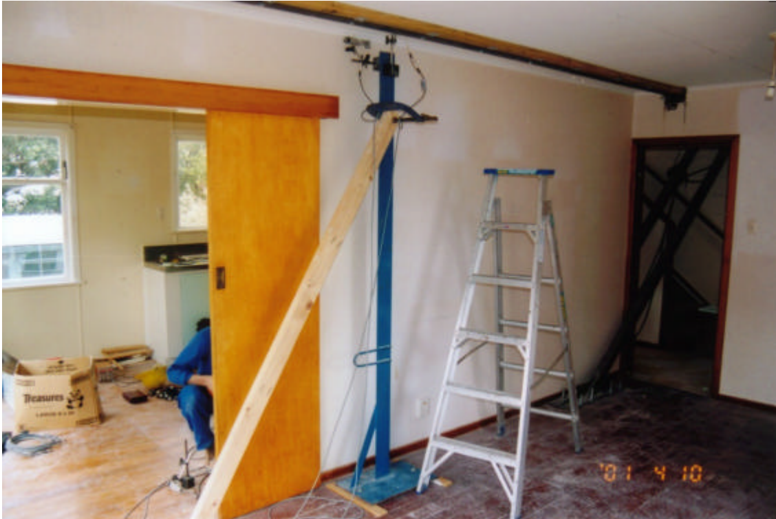
Figure 35: General view of the test wall between the lounge and the kitchen (note that the load application is through the doorway at the right end of the photograph)
