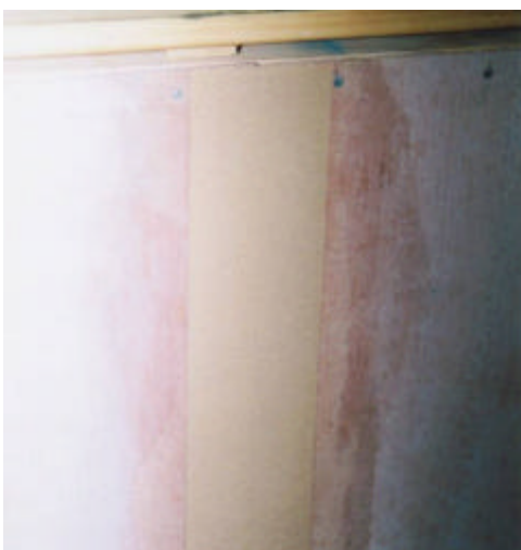
Figure 5 Filled joint between fibre cement sheets
