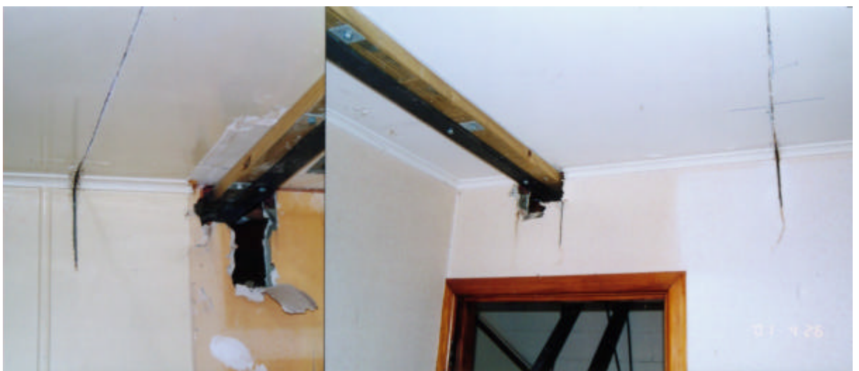
Figure 41: Photographs of the kitchen (left side) and the lounge (right side) showing the cut through the top plate
