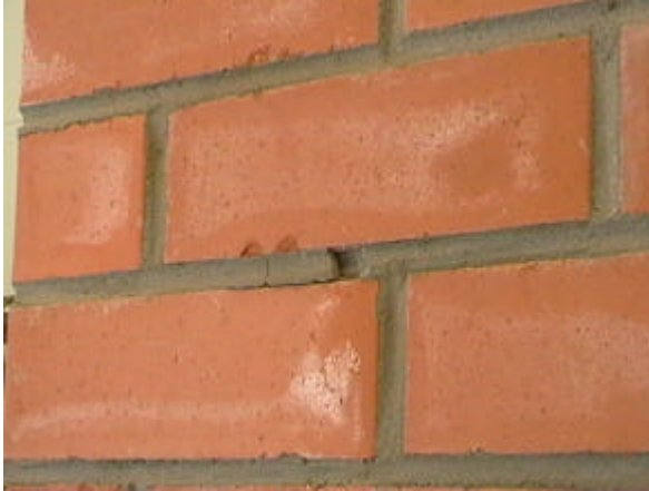
Figure 25: Section of mortar punched out by tie
