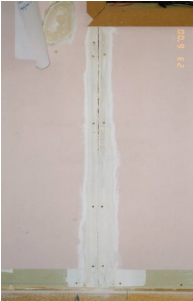
Figure 7: Painted gypsum plasterboard joint prepared for stopping after 15 mm displacement cycles
