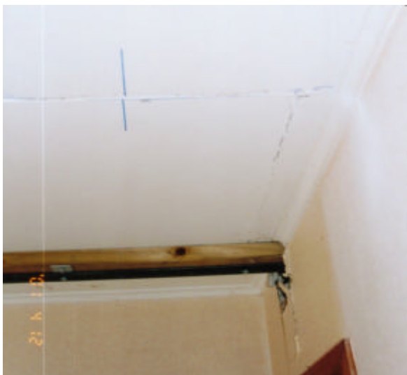
Figure 38: Ceiling misalignment and joint opening
