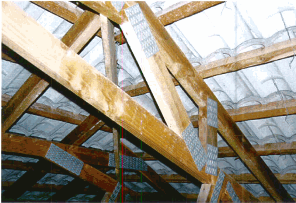
Figure 11: House Roof space.
