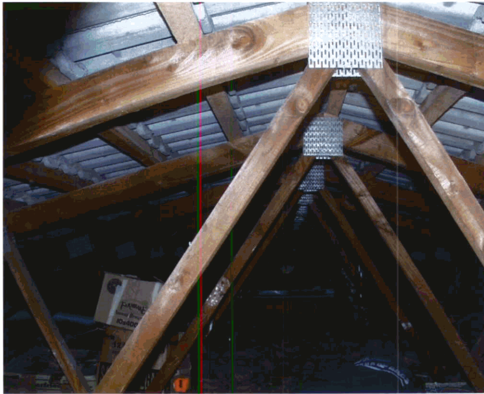
Figure 3: House 001 Roof Space.
