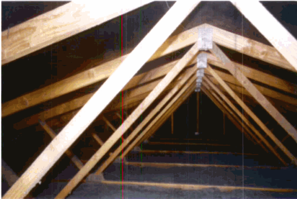
Figure 21: House 007 Roof Space.
