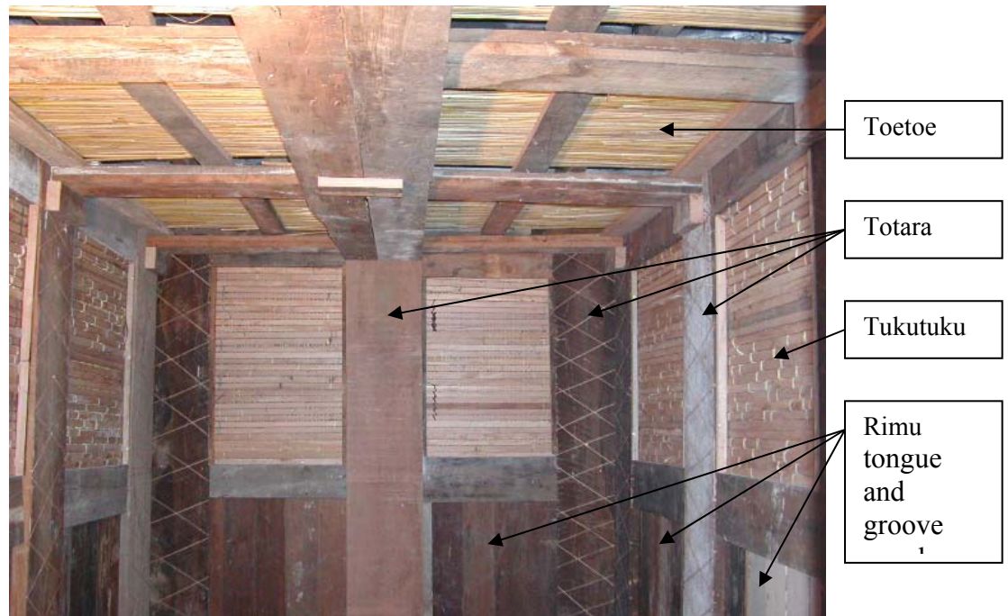
Figure 10-4: Full-scale fire test construction
