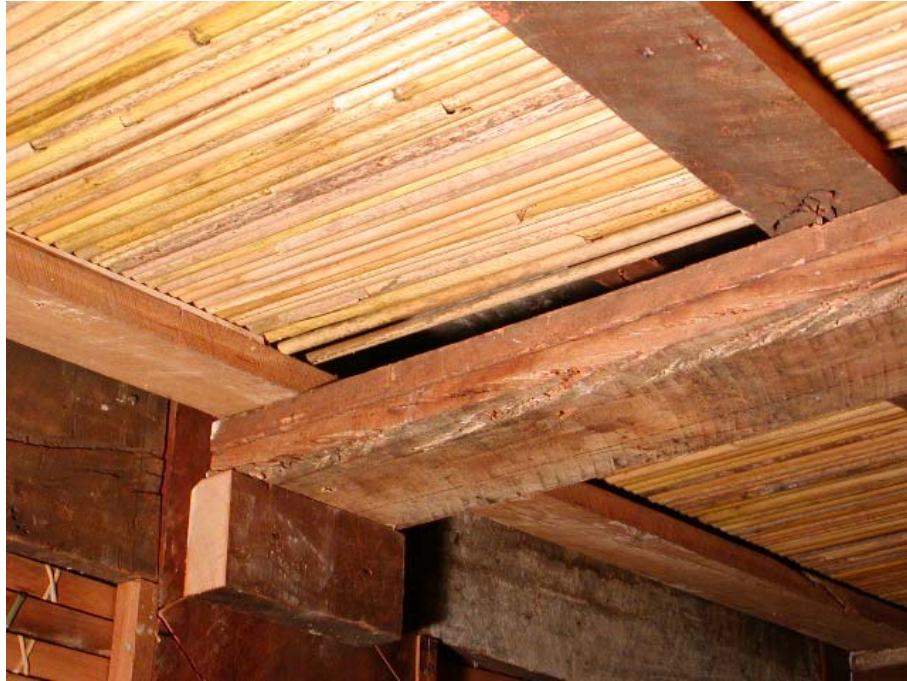
Figure 10-6: Ceiling linings - toetoe and rimu rafters
