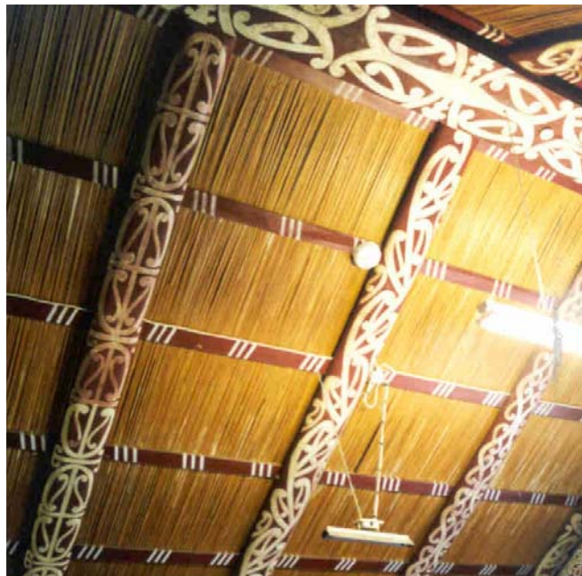
Figure 8-6: Internal ceiling linings
