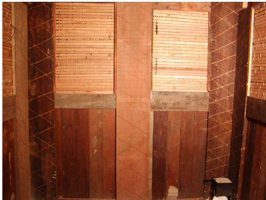
Figure 10-5: Traditional wall linings – tongue and groove, tukutuku and replica carvings
