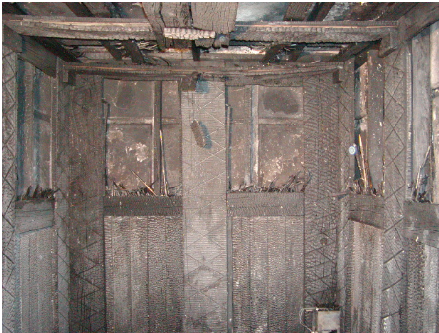
Figure 10-10: Fire test conclusion
