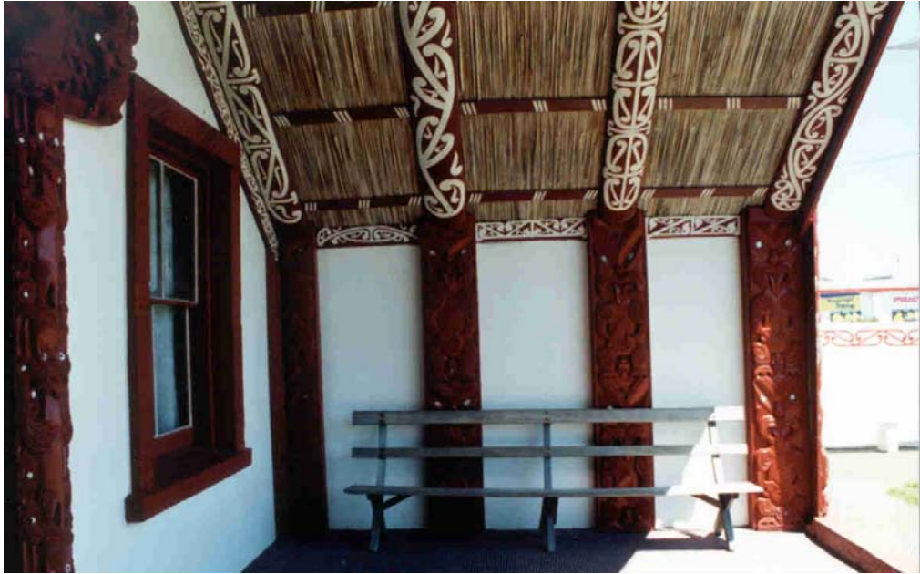
Figure 8-5: Ceiling lining of porch – toetoe thatched together
