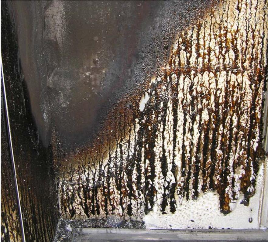
**Figure 13: Ponding of molten EPS at the bottom of cavity**
