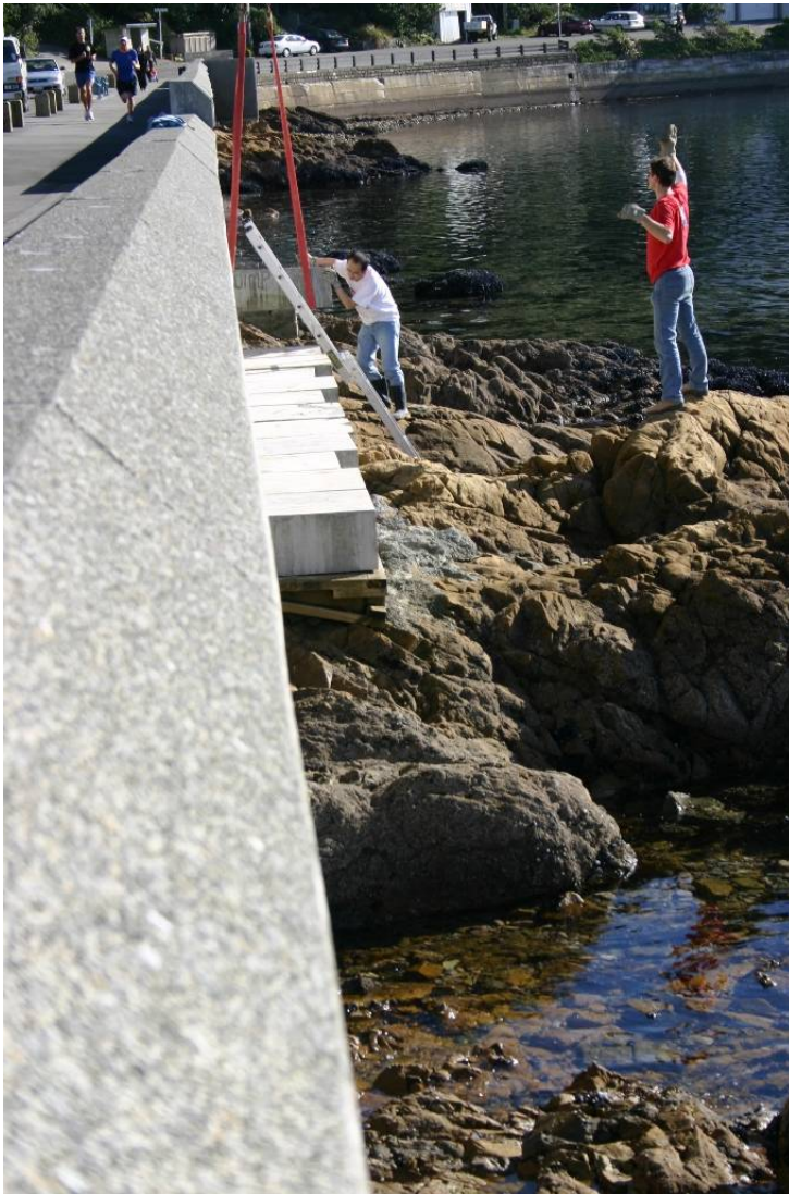
Figure 8: Installation of concrete blocks on Weka Bay C zone exposure site
