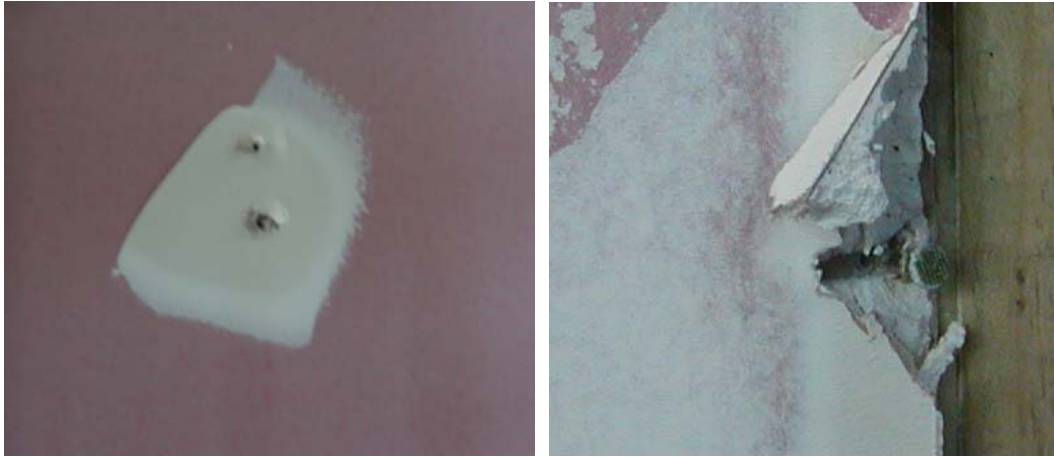
Figure 28: Damage to lining in FR3362A
