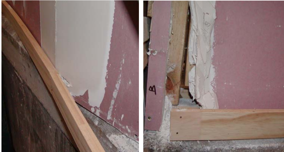
Figure 35: Detachment of skirting board and opening at bottom corner FR3362D
