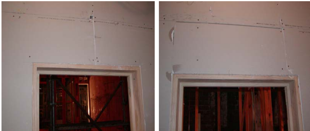
Figure 2: Lining around door frames
