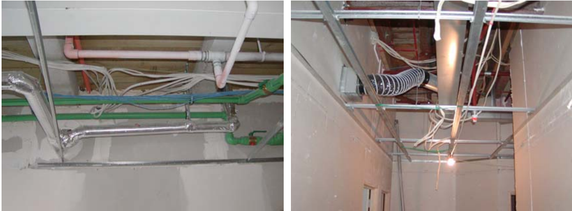
Figure 7: Penetrations above suspended ceiling
