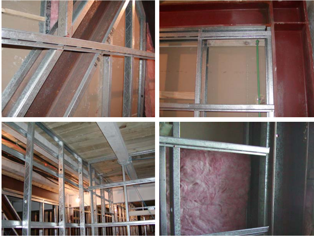
Figure 6: Light steel frame attached to structural steel members and underside of concrete floors
