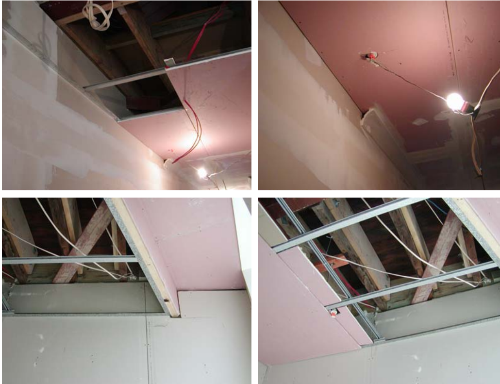
Figure 4: Suspended ceiling ~300 mm below top of wall lining and junction is finished with coving strip and sheet joints are screw laminated
