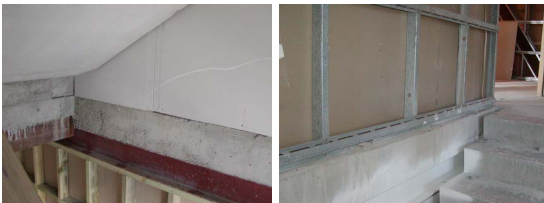
Figure 3: Horizontal joints between floors in stairwells
