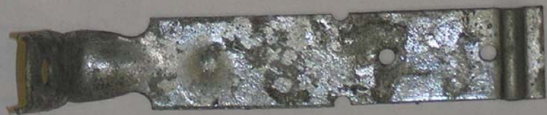
Type B Hot dip galvanised tie for 90 series veneers
