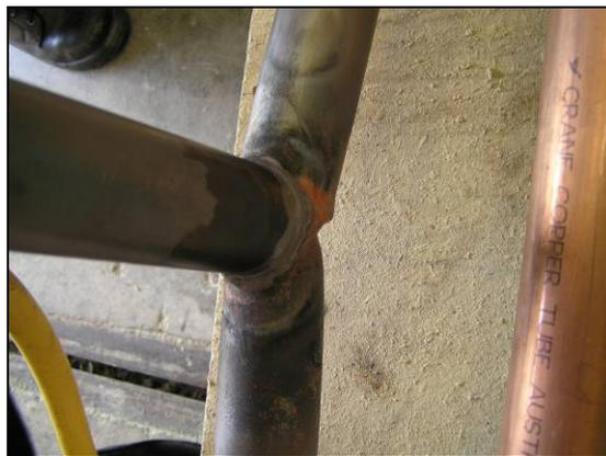
**Figure 20. Kinking of a copper pipe at 'T' joint.**
