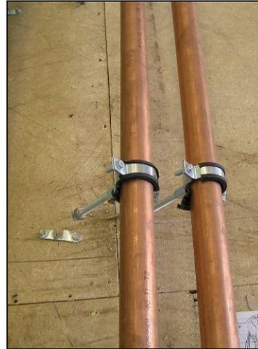
**Figure 21. Total loss of pipe clamp hold-down capacity.**
