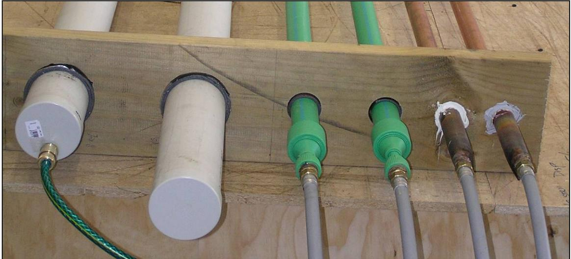
**Figure 7. Fire collars and fire insulation at timber board simulating floor.**
