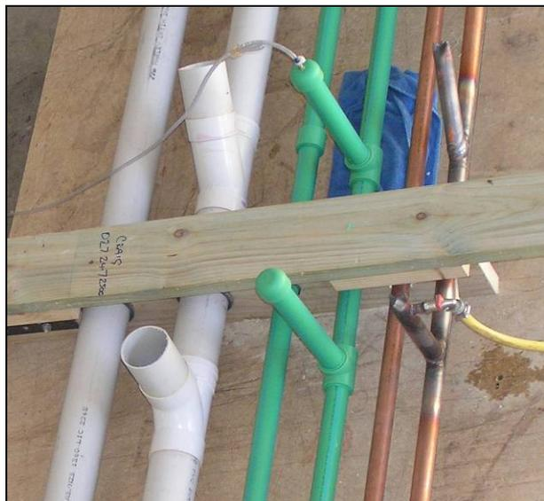
**Figure 6. Pipe 'T' and 45° joints.**
