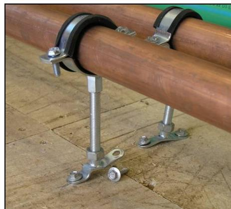
**Figure 17. Pipe clamps losing part of the hold-down fixings.**
