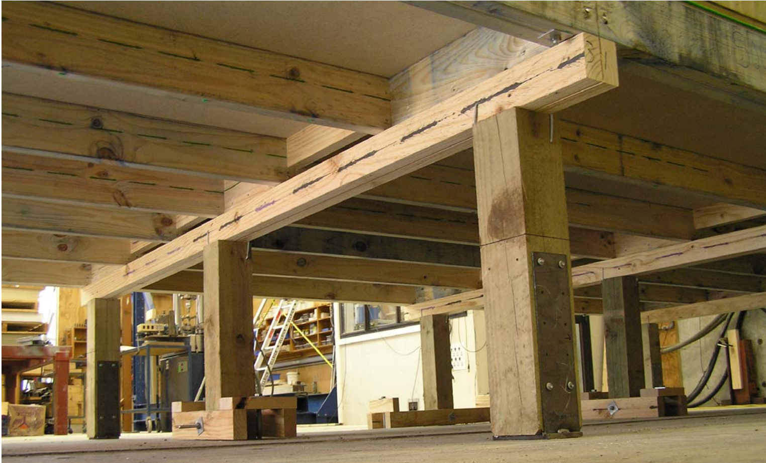
Figure 1. General view of foundation framing.
