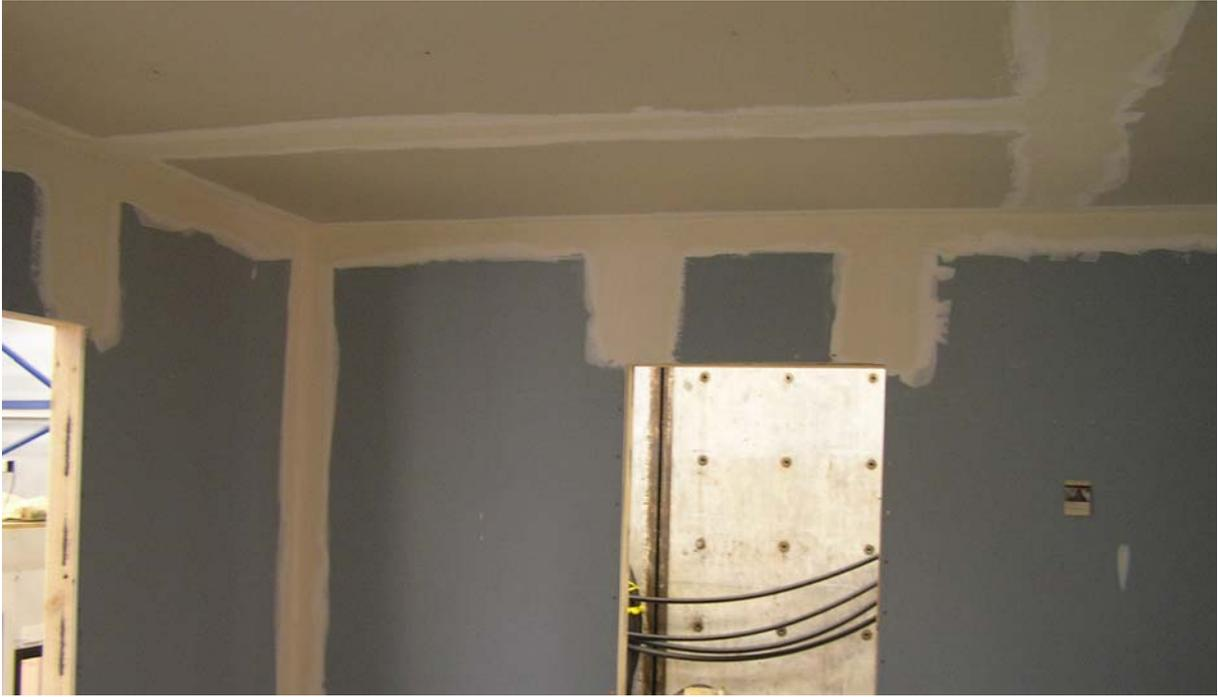
**Figure 11. Photograph of Room 2 interior plastered joints**
