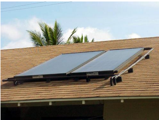
A flat plate collector (cylinder is within building)
