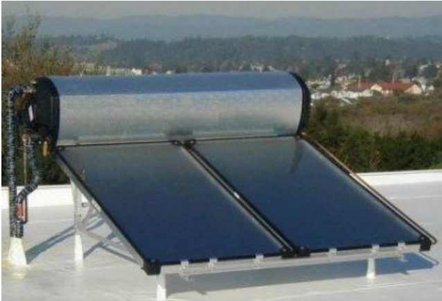
A flat plate thermosiphon system
