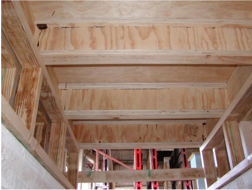
Figure 48. Photograph during construction of Pilot Fire Test Specimen 1
