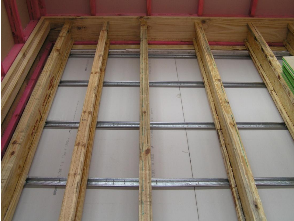
Figure 9. Photograph of the basic floor taken during construction
