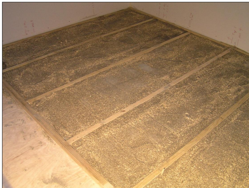
Figure 20. 45 x 45 mm thick batten frame with sand/sawdust mix infill
