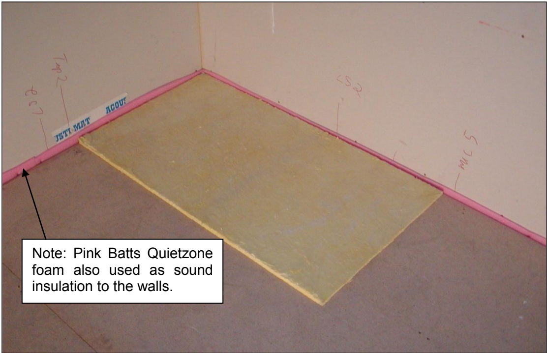
Figure 25. 13 mm fibreglass sound-suppressing layer
