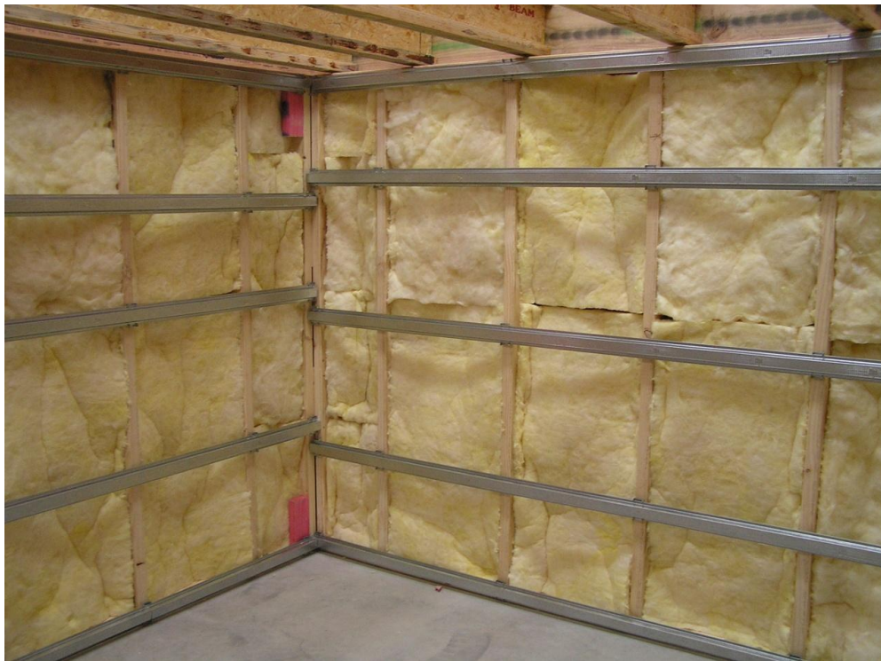
Figure 8. Photograph of exterior walls of the acoustic chamber taken during construction showing the acoustic absorption and furring channels connected to the frame with RSIC-1 clips.
