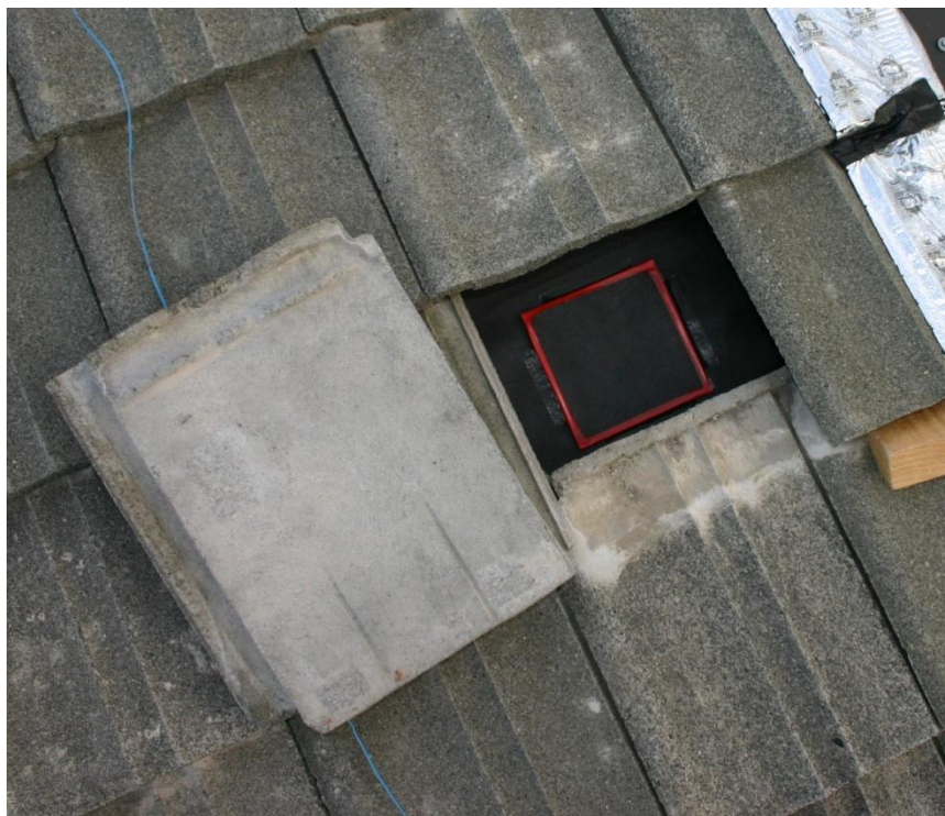
Figure 9. Picture of the condensation apparatus for roof specimens with concrete tiles
