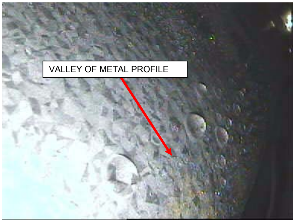
Figure 17: Condensation accumulates near the valleys of the corrugated metal profile
