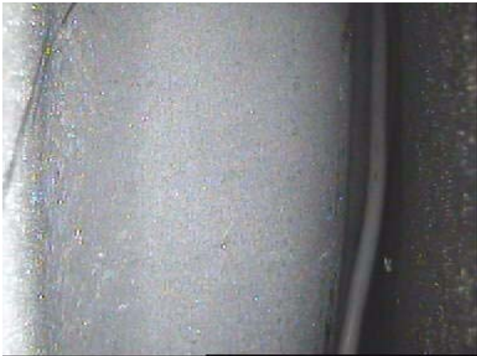
Figure 13: Condition of the cavity 30-40 minutes after the start of the dry ice experiment. The underside of the metal cladding is covered by a thick layer of frost
