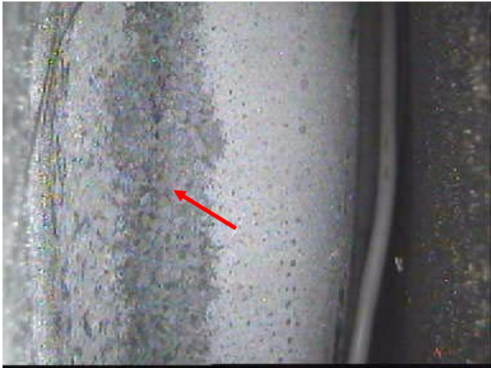
Figure 14: After removing the dry ice, the layer of frost starts to melt nearly immediately
