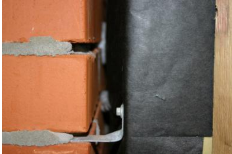
Figure 22: Cavity of Brick Veneer Wall (D4863a)
