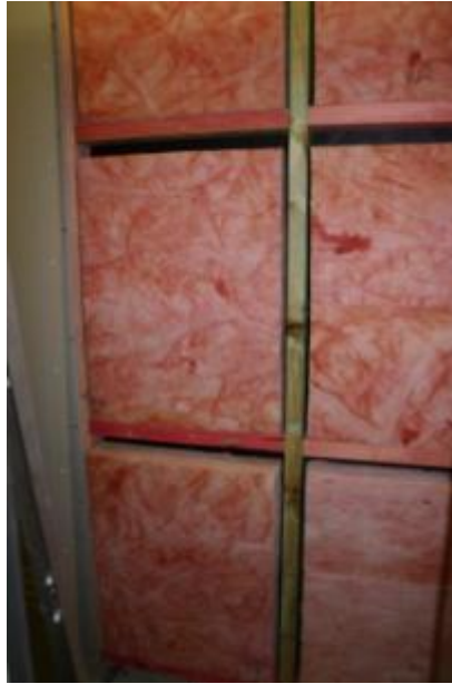
Figure 21: R 2.8 glasswool insulation fitted with 3% gaps at side and 6% gap at the top of each frame cavity (D4862b)
