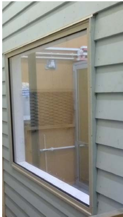
Figure 10. View of window in weatherboard clad walls in the Hamilton test
