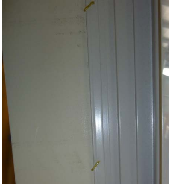
Figure 11. Typical reveal-to-window frame stapling used in the Hamilton test
