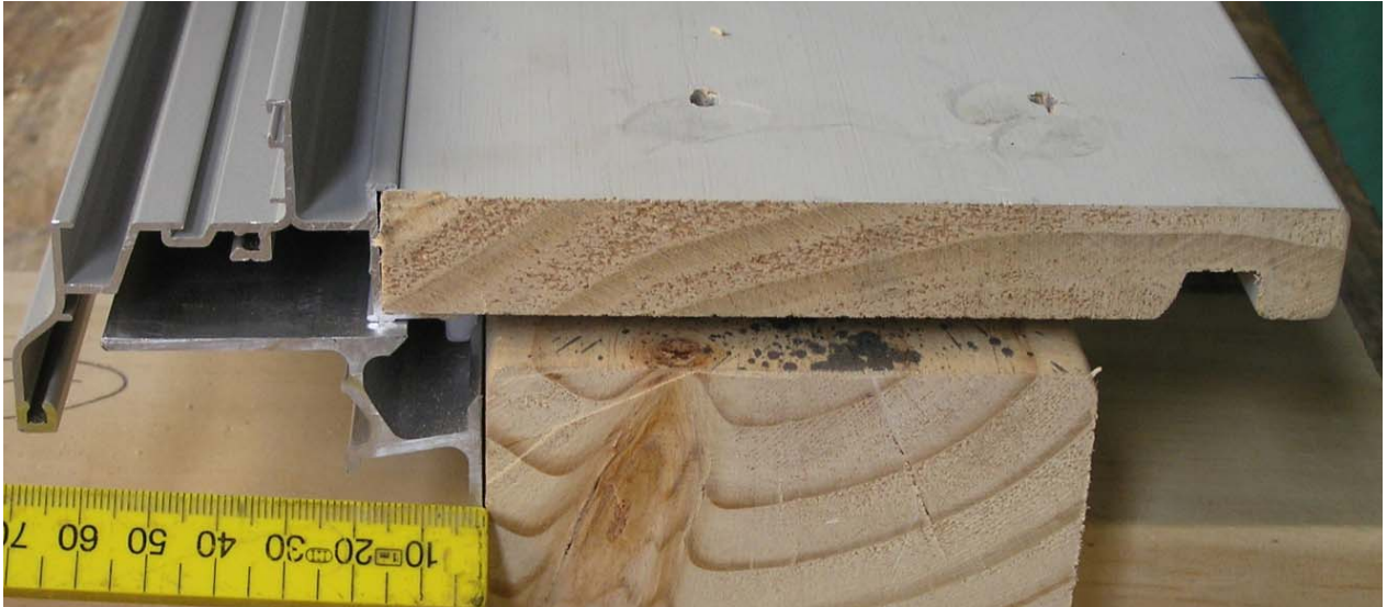
Figure 22. Photograph taken during installation of joinery to the dummy sill
