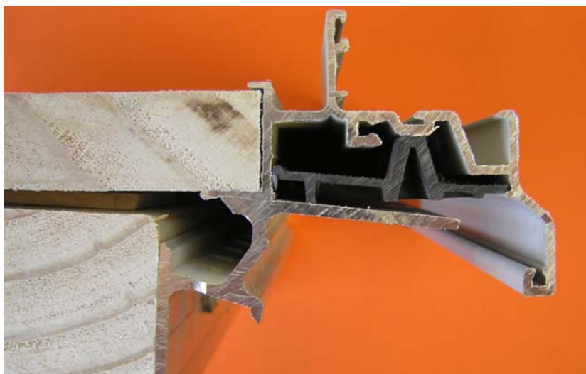
Figure 24. Window support block (black) in as-used position
