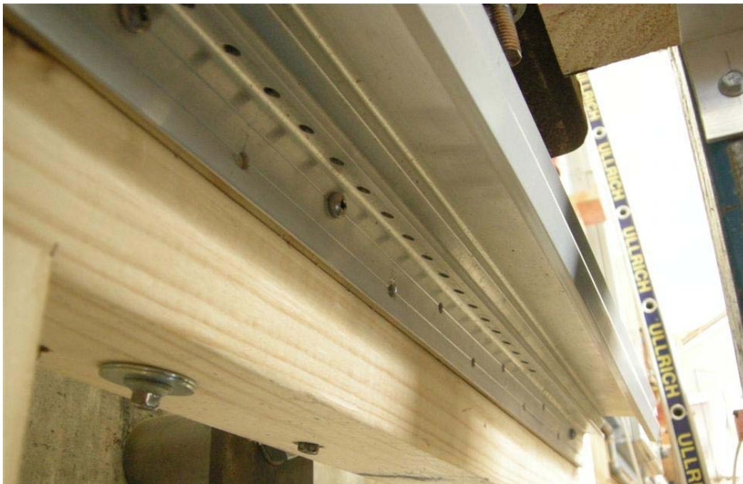
Figure 39. Screws fixing Wanz bar to the sill trimmer at test completion – no apparent pull-out
