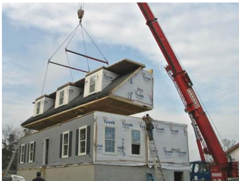
Figure 2: A modularised home being assembled onsite by crane
