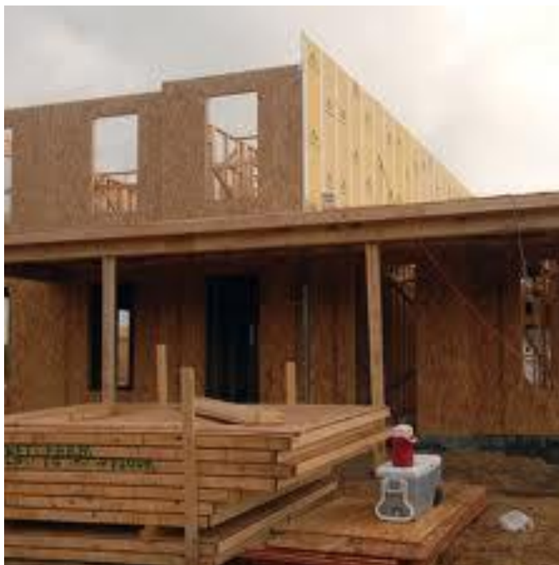
Figure 10: A panelised home under construction in the USA
