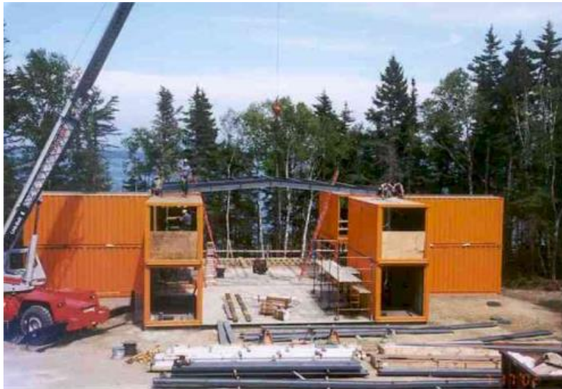
Figure 1: A hybrid prefabricated dwelling under construction, utilising shipping containers
