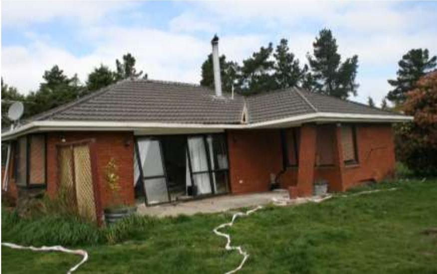
**Figure 9. House severely damaged by differential ground settlement and lateral spreading**
