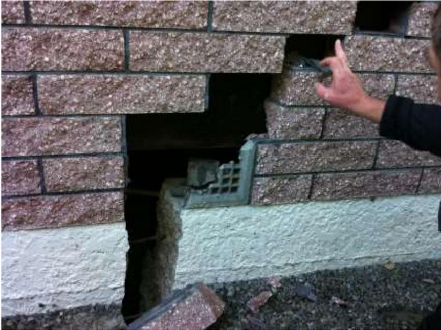
**Figure 10. Example of reinforced concrete perimeter foundation pulled apart by spreading ground (note reinforcing bar crossing gap in foundation)**
