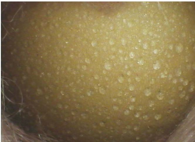
Figure 10. Wall 8 – widespread condensation as in year 1.
