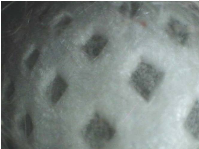
Figure 12. Wall 9 – no condensation visible in part 1 of year 2.
