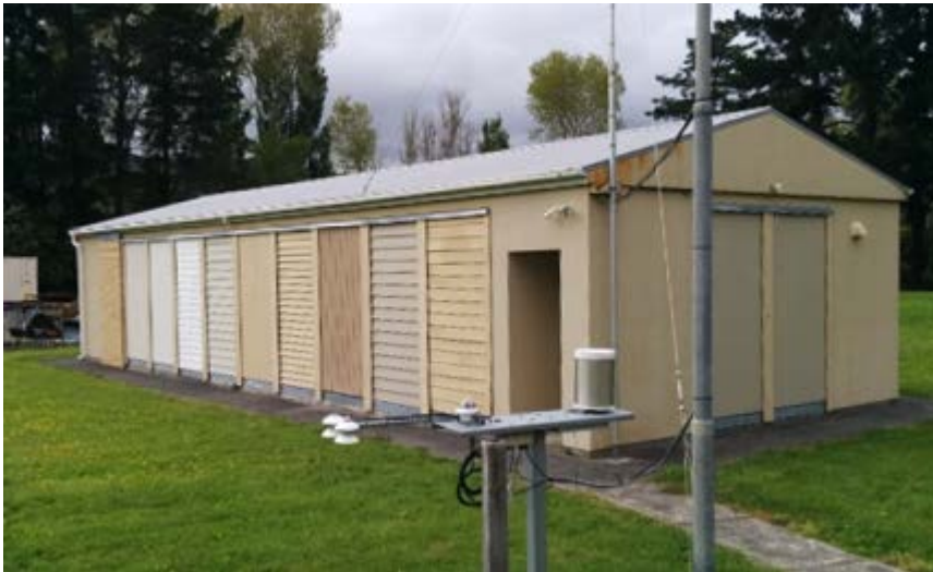
Figure 3. Test building on the BRANZ site – weatherstation shown in foreground.
