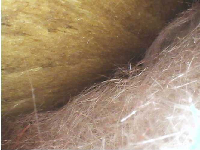
Figure 11. Wall 6 – no condensation visible on plywood.
