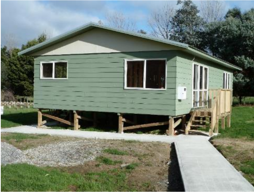
Figure 4. BRANZ ventilation research building – before enclosing subfloor.
