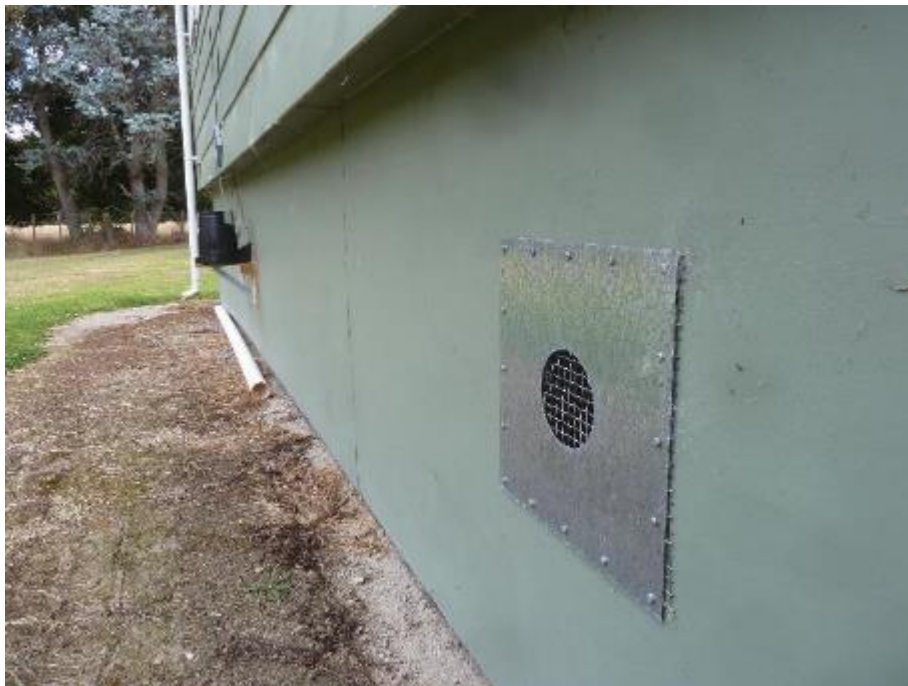
Figure 6. Subfloor vent.
