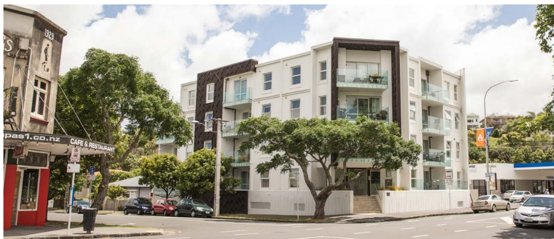
Photo 7. Example of a 3-storey apartment building.
