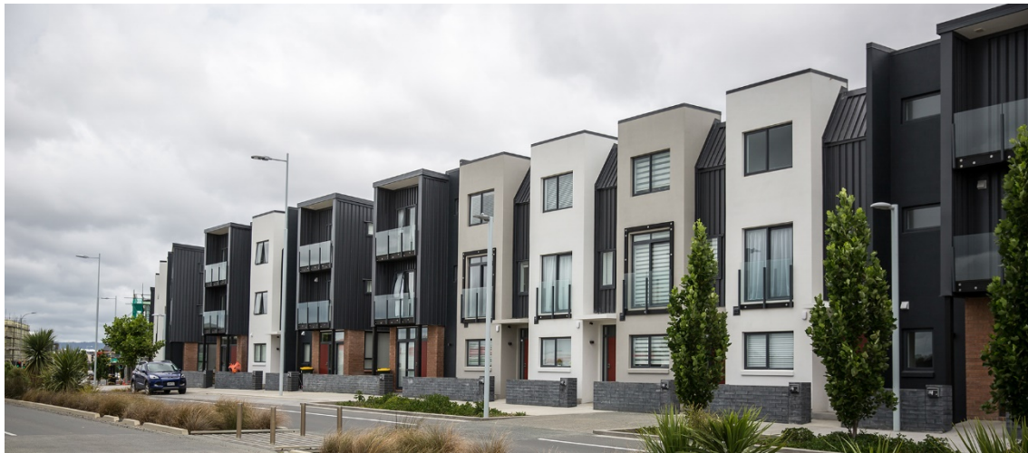
Photo 5. Example of a 3-storey terraced house.
