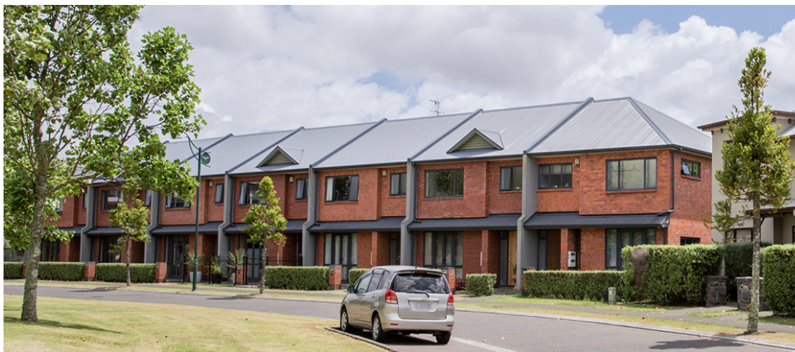
Photo 4. Example of a 2-storey terraced house.
