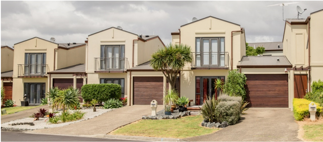
Photo 3. Example of 2-storey attached duplex.
