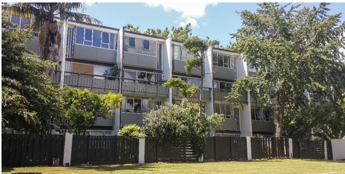
Photo 6. Example of a 4-storey terraced house,
