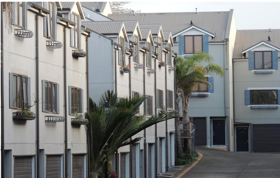
Figure 6. 3-storey terraced MDH.
