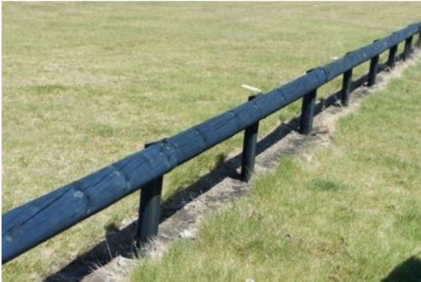
Figure 66. An example of wood discolouration noticed in an area with strong geothermal influences (south of Sulphur Bay).
