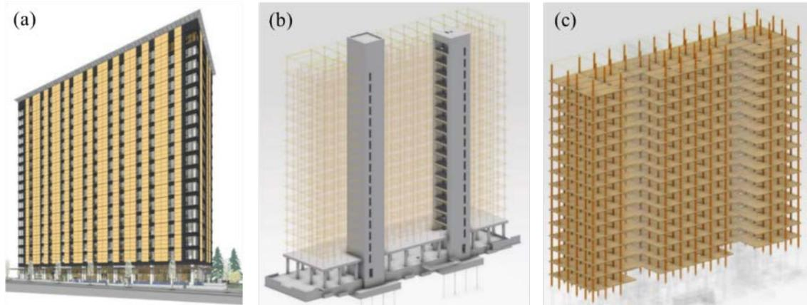
**Figure 26. Brock Commons, a timber-based hybrid 18-storey building in Canada: (a) architectural concept; (b) RC first storey (podium) and core walls; (c) timber frames.**
