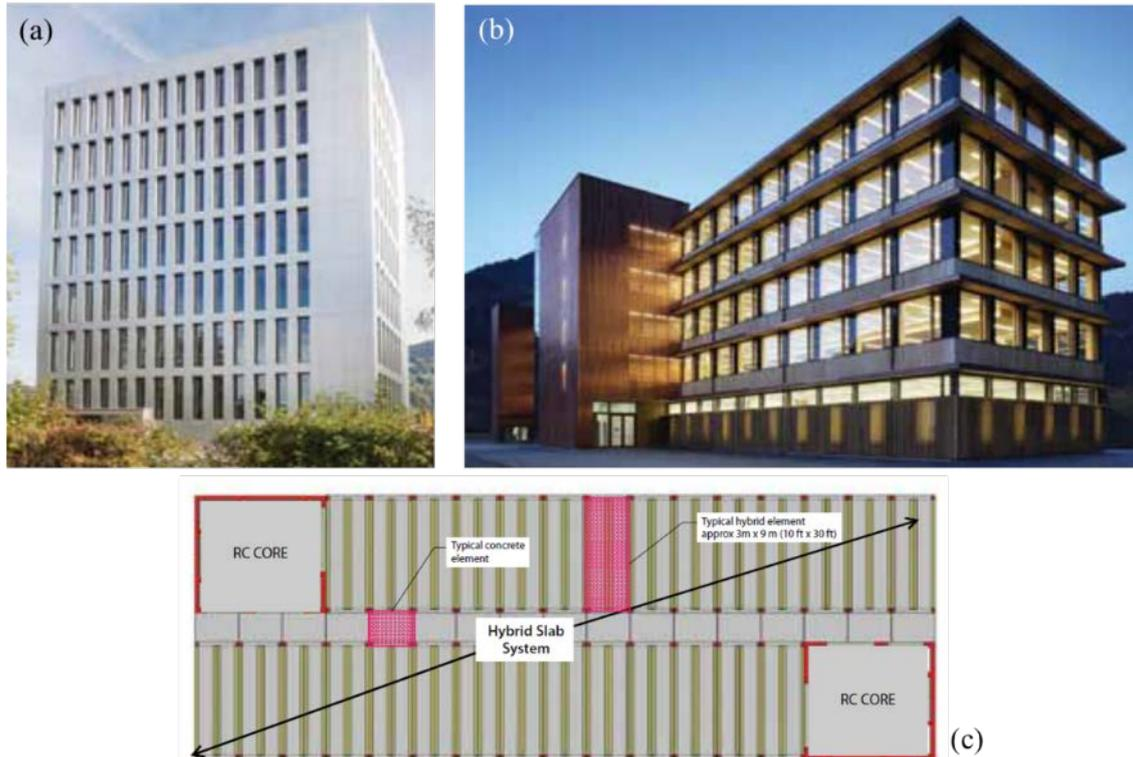
**Figure 25. Hybrid construction in Austria: (a) 8-storey prototype building (LCT One, Dornbirn); (b) 6-storey office building (LCT Two, Montafon); (c) structural layout of modified prototype to account for seismic actions.**
