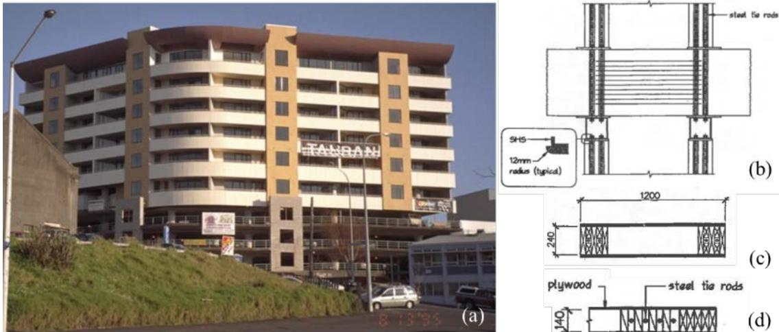
**Figure 21. Gulf View Towers hybrid building: (a) overview; (b) beam-column joint details; (c) plywood box column cross-section; (d) plywood box wall cross-section.**
