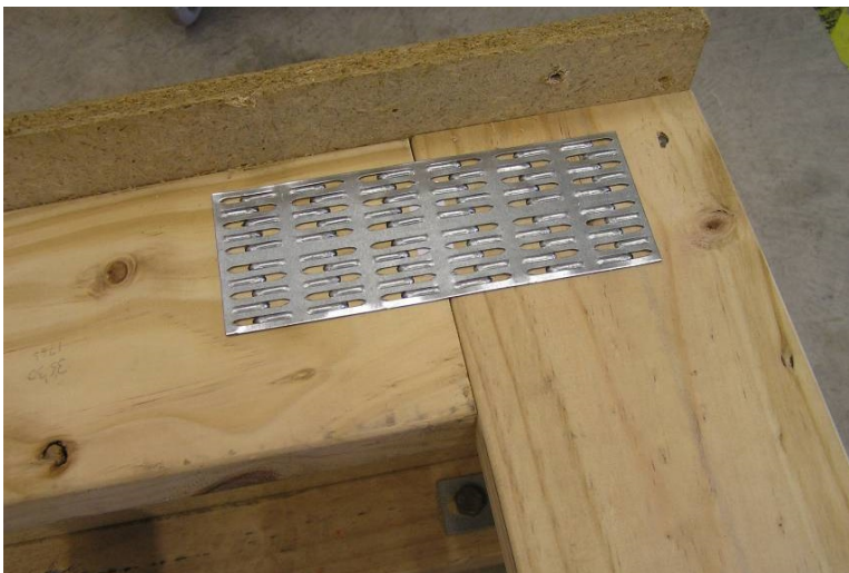
Figure 27. Mitek 6T10 Tylok connector at corners of diaphragm.
