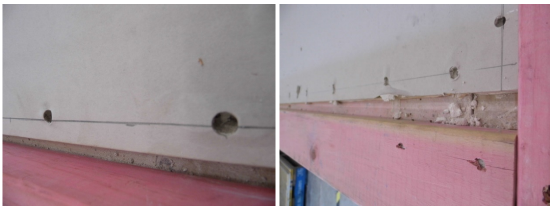
Figure 33. Damage associated with screw failures.
