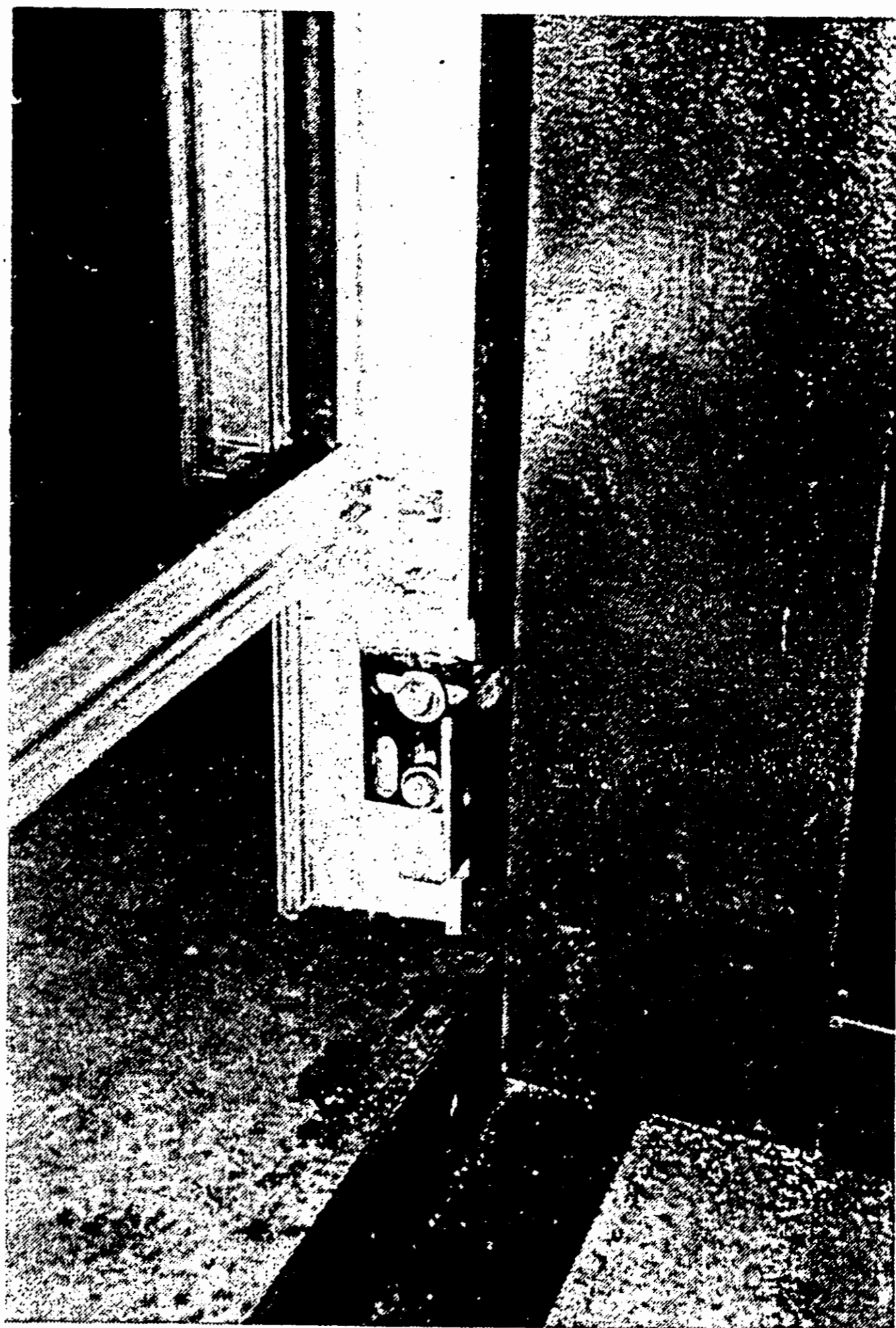
Figure 5b : Fixing of mullion to channel as viewed from the interior
