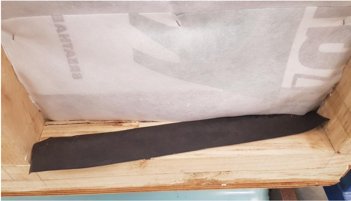
Figure A5. Close-up view of the pulled-out strip of kraft paper tucked between the framing and the underlay. This image was taken after the test.
