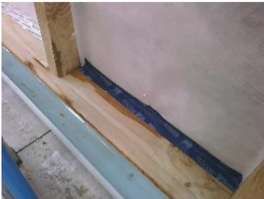
(j) Water was transferred to framing
