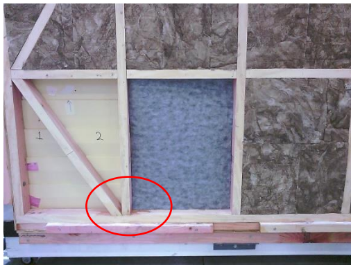
(a) Water was transferred to framing
