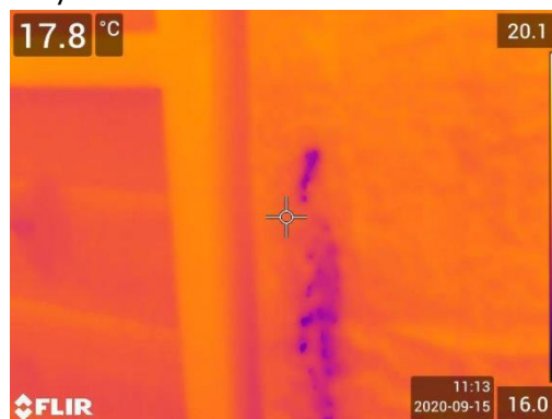
Figure 10. Walls insulated with drainage plane mesh and underlay.
