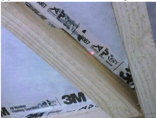
(l) Water was transferred to framing
