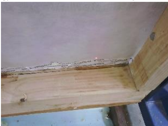
(k) Water was transferred to framing
