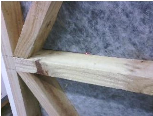
(c) Water was transferred to corner of diagonal bracing
