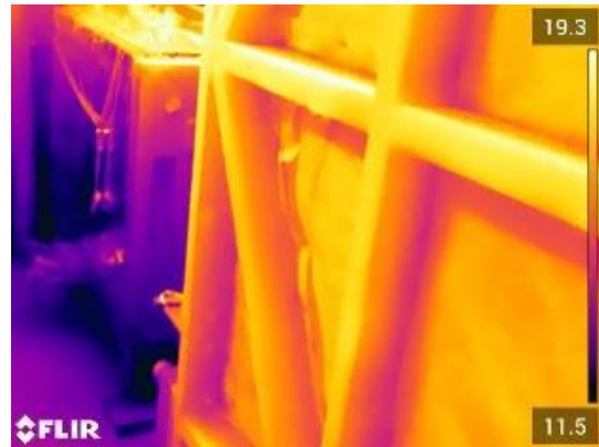
(a) Strip of synthetic underlay tucked between framing and back of cladding
