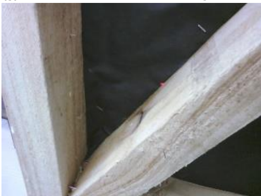
(h) Water was transferred to diagonal bracing
