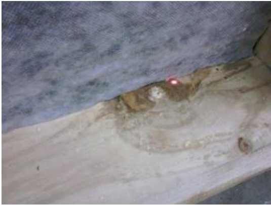
(b) Close-up view – water was transferred to bottom plate with knot in it
