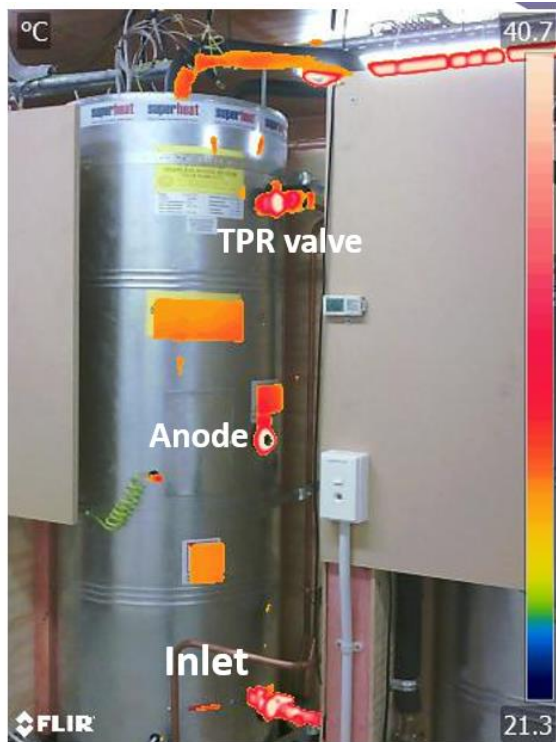
Figure 4. Hot water cylinder with thermal image overlays of connection points to the cylinder and temperature scale on right-hand side.
