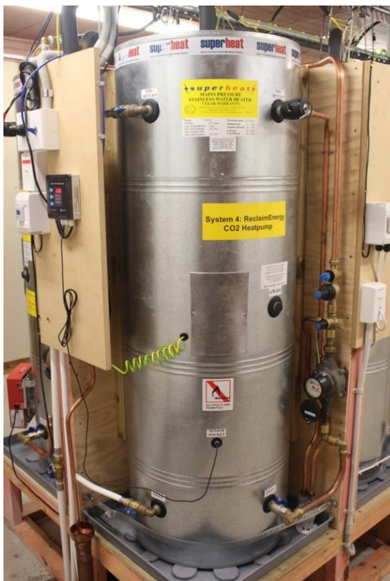
Figure 9. Cylinder used with the Reclaim Energy CO 2 heat pump system.
