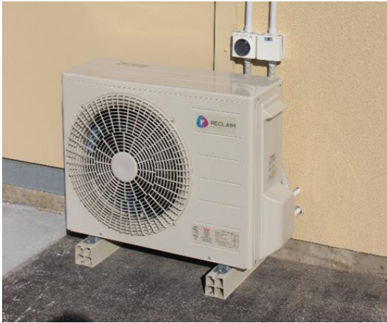
Figure 10. Reclaim Energy CO 2 outdoor unit.
