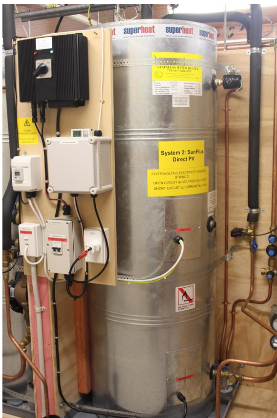
Figure 7. Sun Flux controller (black unit) top left.
