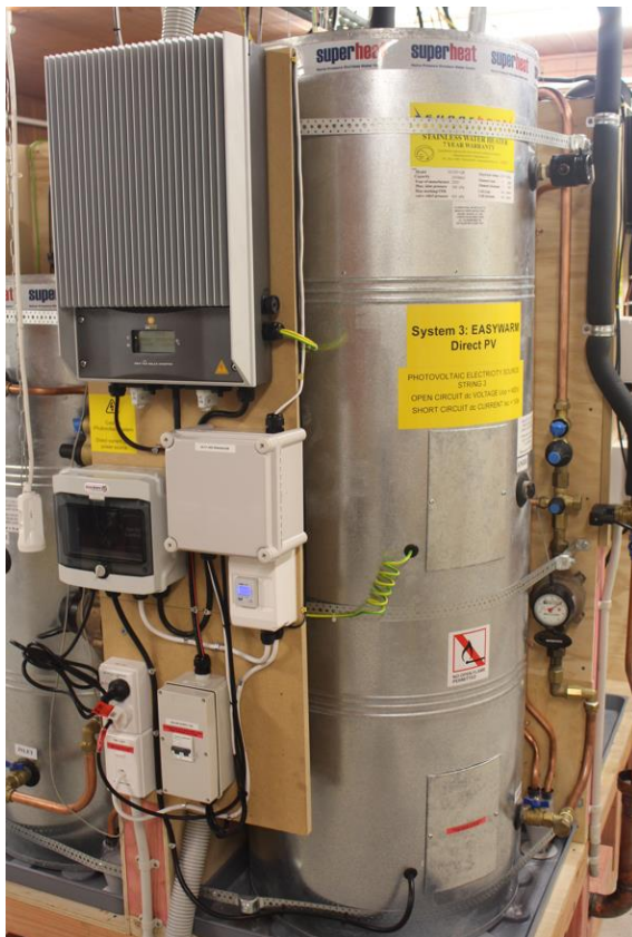
Figure 8. Easy Warm system with EnaSolar inverter.
