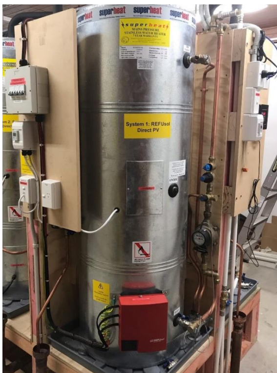
Figure 6. REFUSol controller (red unit) with DC cables from the three PV strings connected to the unit.
