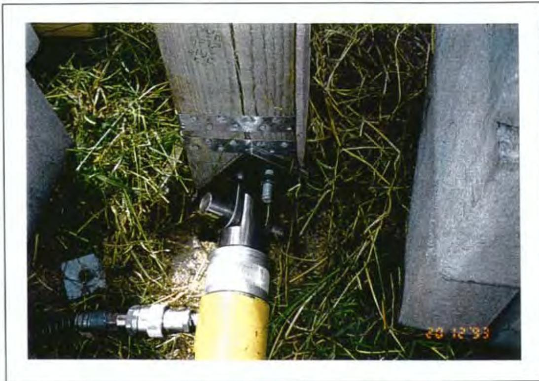
(c) Jacking Location on Shear Piles
