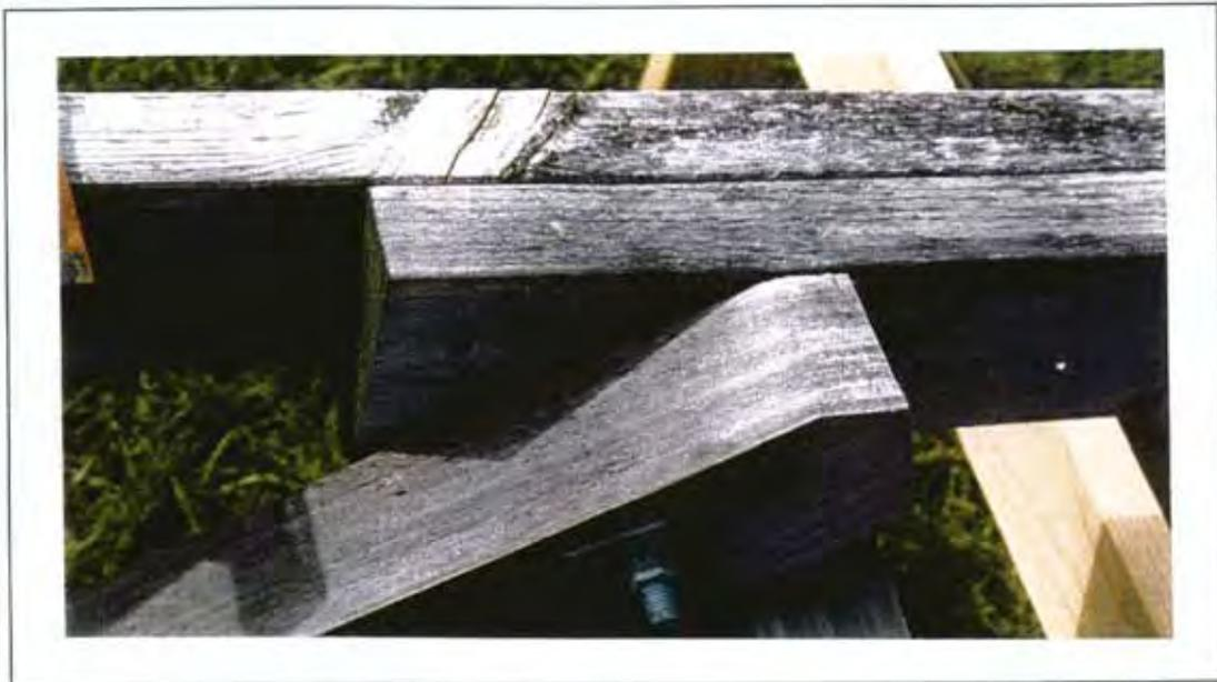
(b) Connection of Brace to Joist (Short length packer sandwiched between)
