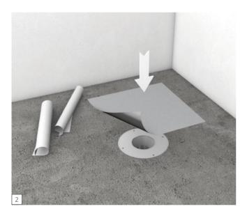
Following the respective manufactures floor drain installation instructions, now apply the one-sided self adhesive sealing gaiter to the drain and surrounding surface.
