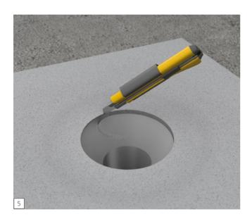
For "floor drains with clamping ring", the floor sealing gaiter is cut so precisely that the cuff overlaps the interior of the drain by a few millimetres. The cuff must not sit under the clamping ring of the drain which will be installed later.
