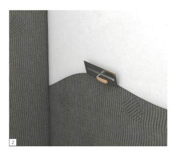
The tile adhesive should be applied to the full surface using a notch trowel (4 or 6 mm grooves).
