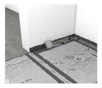
Seal corner and wall-to-floor joints with wedi sealing tape and wedi 620 sealant. The sealing tape should be applied centrally on the joint. Sealing corners, sealing tapes or moulded parts are placed on the fresh adhesive sealant layer and pressed into place (e.g with a trowel, float or pressure roller) so that the sealant is pushed out of the sides. The excess material is removed smoothly with a trowel. Creases and distortions should be smoothed out and pressed down.
