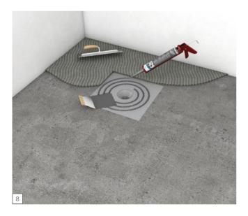
Apply the tile adhesive on the prepared surface with a 4 or 6-mm square trowel. If required, the surface must be primed. This should be done prior to the installation of the floor sealing gaiter. Once primer has cured sealing gaiter can be installed and adhesive applied.
